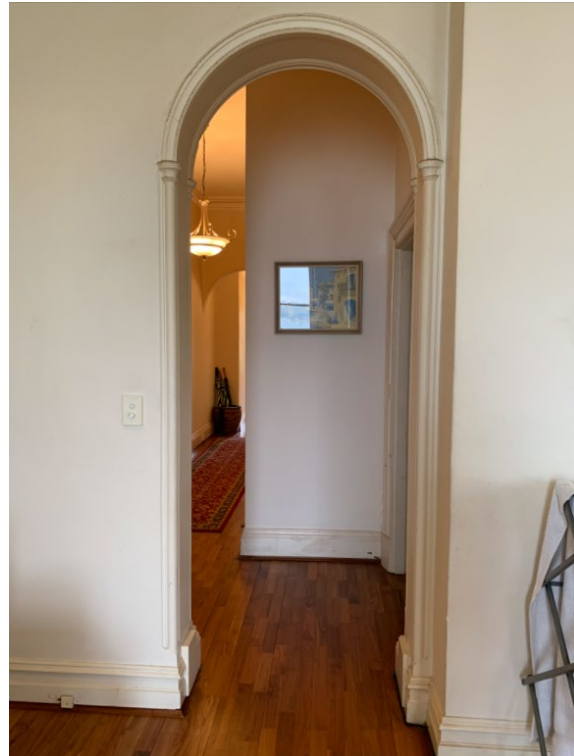
Figure 8: Staff moulds to the living room arch reveals, Flat 1. (Source: WMC Officer, October 2020)
