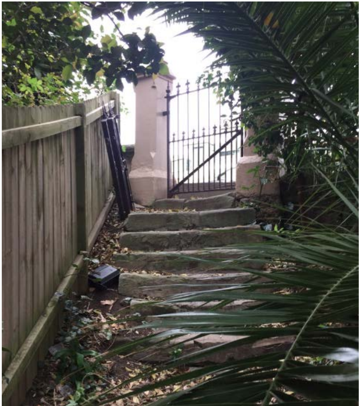
Fig. A2.6 The sandstone block entry steps leading to the eastern entry porch, do not appear to be in use, probably due to their settlement and garden growth.
