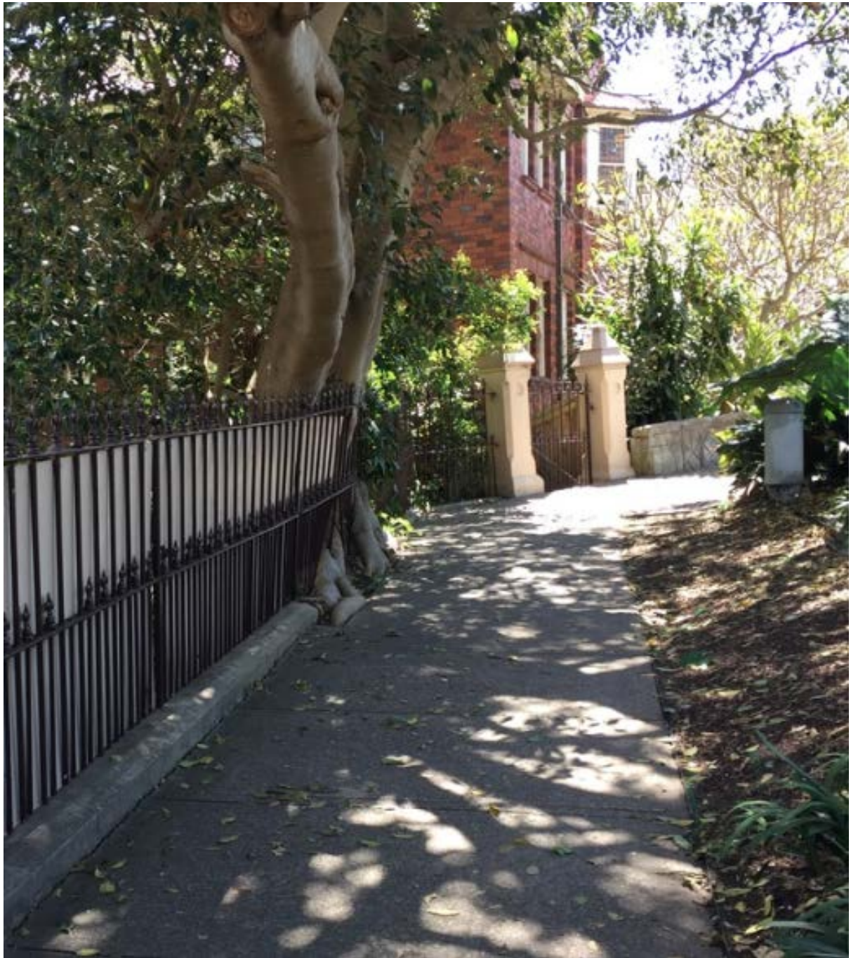
Fig. A2.5 The eastern part of the original wrought iron and masonry palisade with its surviving original eastern gate piers and gate. The fig tree has gradually pushed the fence out of alignment.
