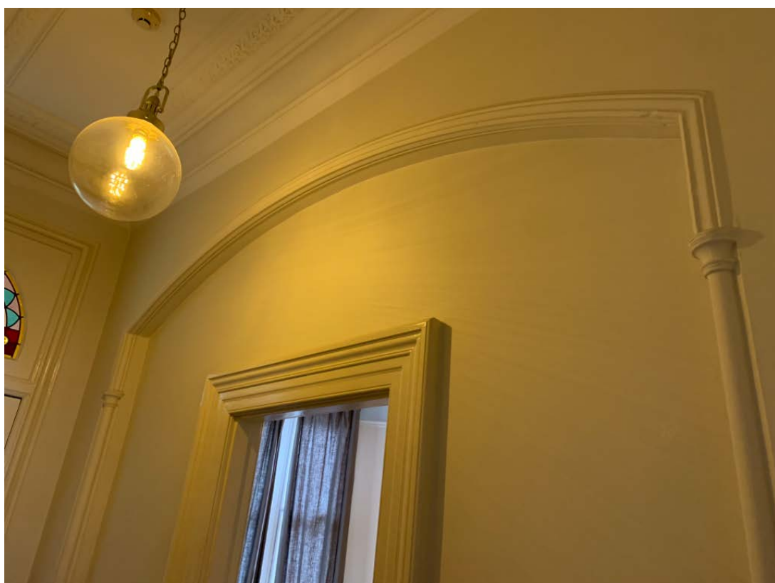
Fig.A2.16 Staff moulds to main hallway blind arch, Unit 3. (Source: K Welfare, October 2020)
