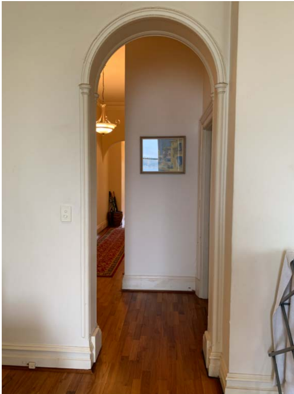
Fig.A2.13 Aesthetic Movement staff moulds to the reveals of the arch to the living room, of Flat 2. (Source: K Welfare, October 2020)
