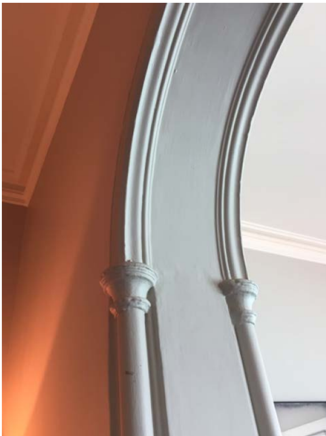
Fig.A2.10 The remarkable Aesthetic Movement staff moulds to the reveals of the arch to the former main bedroom, now living room, of Flat 2.
