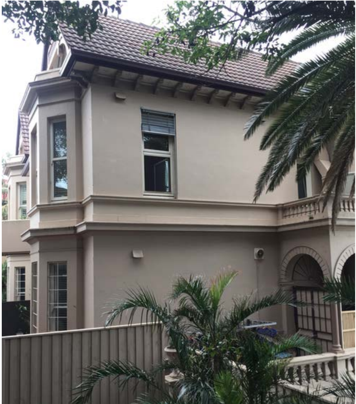
Fig a2.2 The eastern side of the building ; street façade with entry bridge at left, and the former entry porch at right. The heavy, console bracket supported eaves are an example of the building's unusually rich embellishment, as is the round-arched, column-supported and balustered parapet topped porch.
