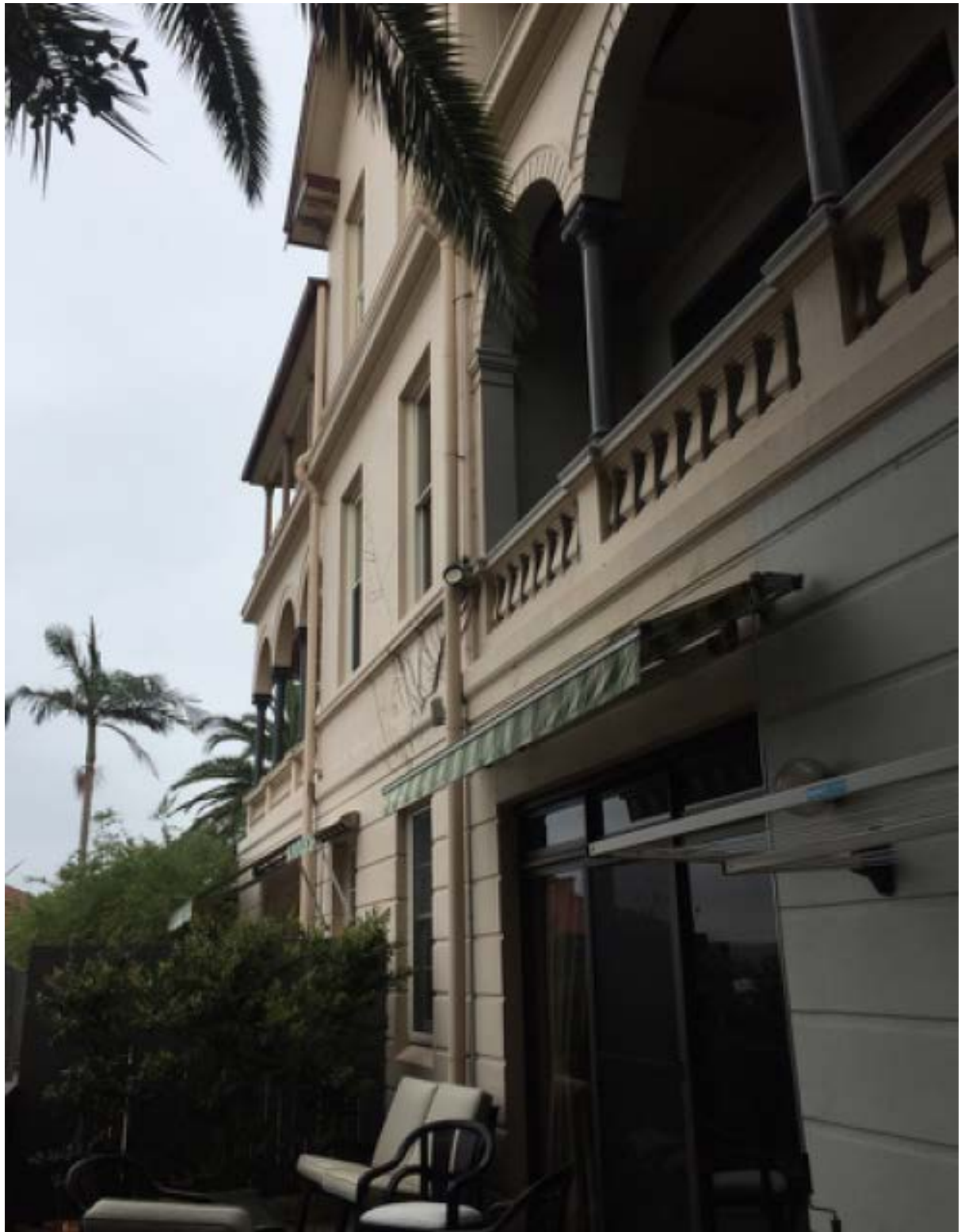
Fig. A2.4 The north, harbour-facing elevation of the building, its principal façade and viewpoint exploiting its original “marine villa” location. Further openings have been made into the rusticated walls of the basement, allowing its flats the use of the close northern setback area left by subdivision.
