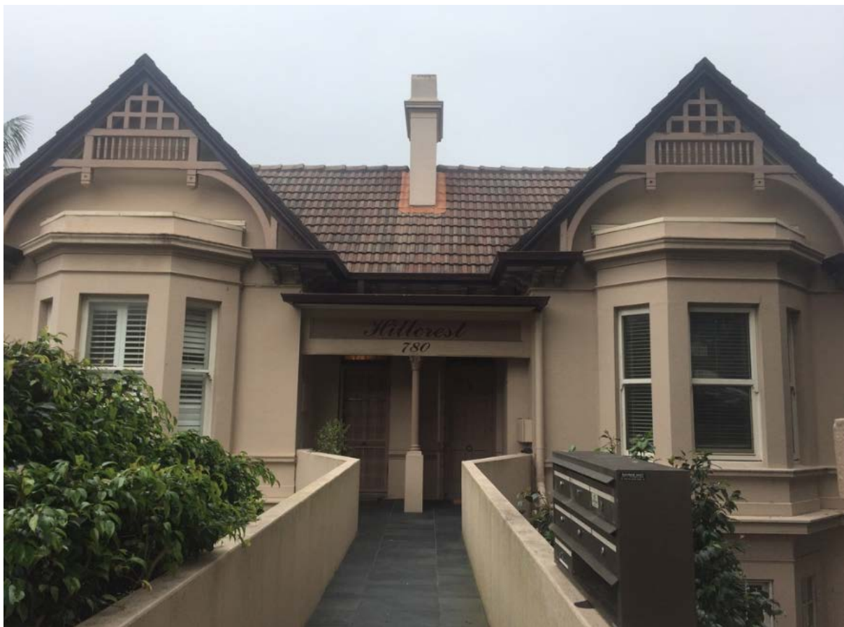
Fig. A2.1 The twin gable presentation of “Hillcrest” clearly reflects its original two dwellings. The concrete entry bridge to the uppermost flats 1 and 2 appears from photographic images to have replaced an earlier bridge probably of timber framed construction. The entries may have been fitted into a re-entrant bay or in place of a balcony. The batted and spindled gable screens are distinctive stylistic touches. The concrete replacement of the slate roof may have caused the loss of detail trim.
