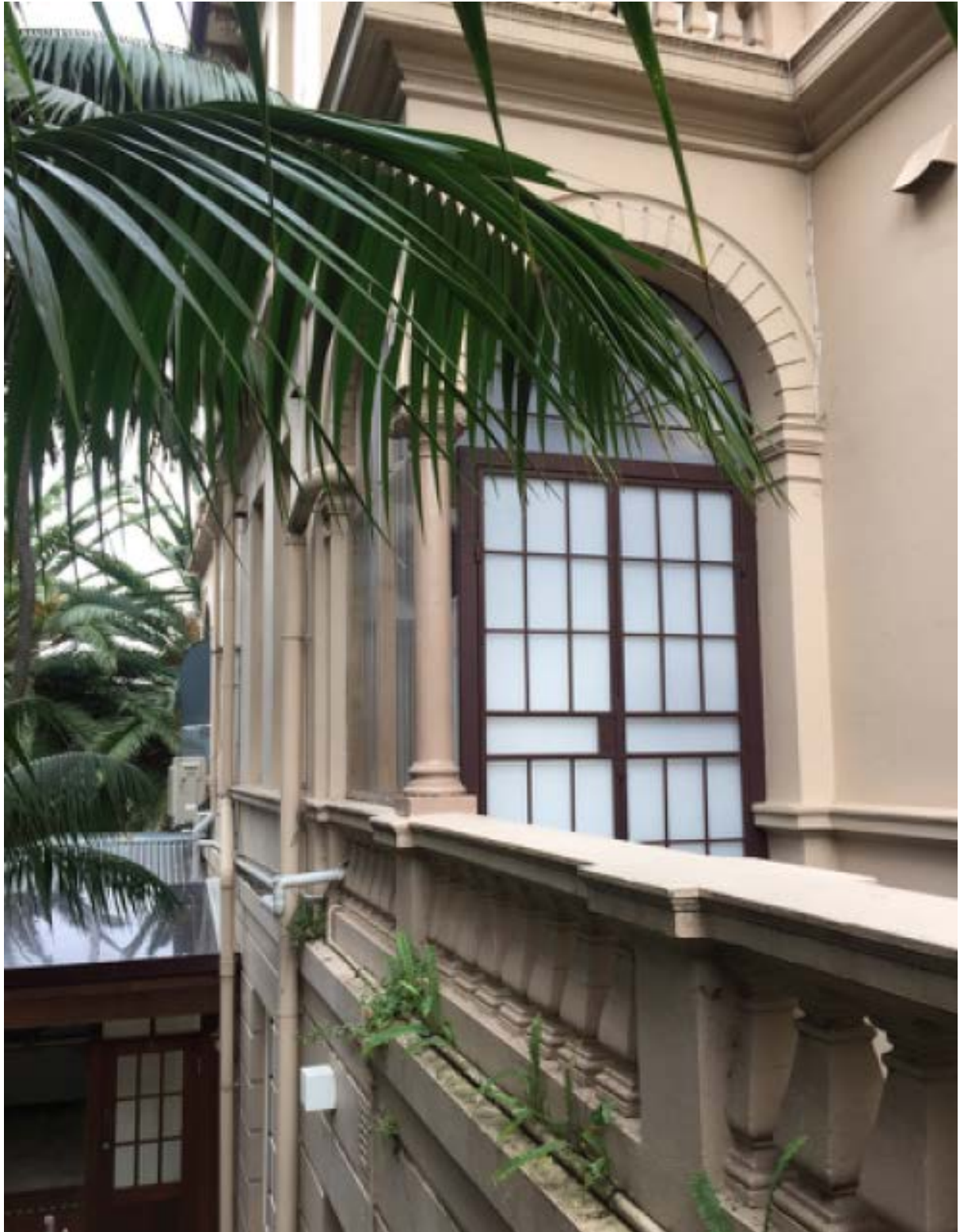
Fig. A2.3 A detail view of the western porch, now the entry to Flat 3 which has been pragmatically enclosed for security and privacy. The side extensions to Flat 5 in the former basement level are visible at lower left. Surface mounted plumbing and services are not helpful to presentation but can be reconsidered.
