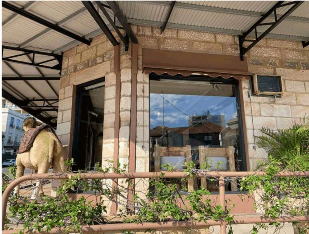
Figure 52: Glenmore Road frontage, including underside of awning and downpipe detail, and intrusive services such as air conditioning units, May 2021.
