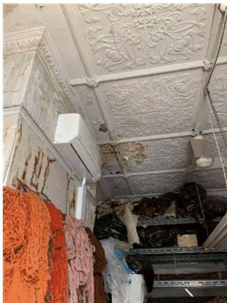
Figure 59: Level 2 decorative ceiling and cornice elements, with water damage visible
