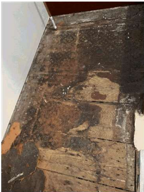
Figure 69: Multiple floor finishes visible on the southern stair landing
