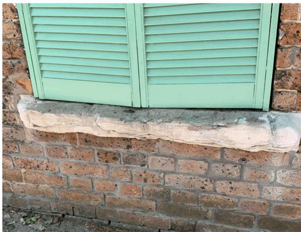
Figure 39: Weathered sandstone windowsill of 545 Glenmore Road, March 2020.
