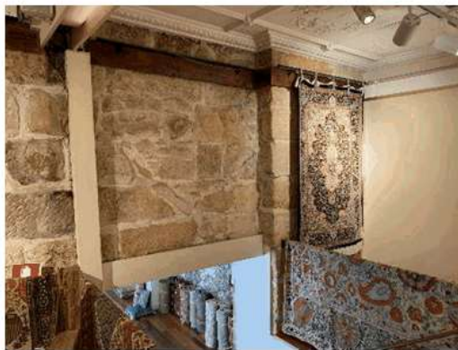
Figure 64: First floor level exposed sandstone walls, with gallery rug display rails affixed to the top part of the wall
