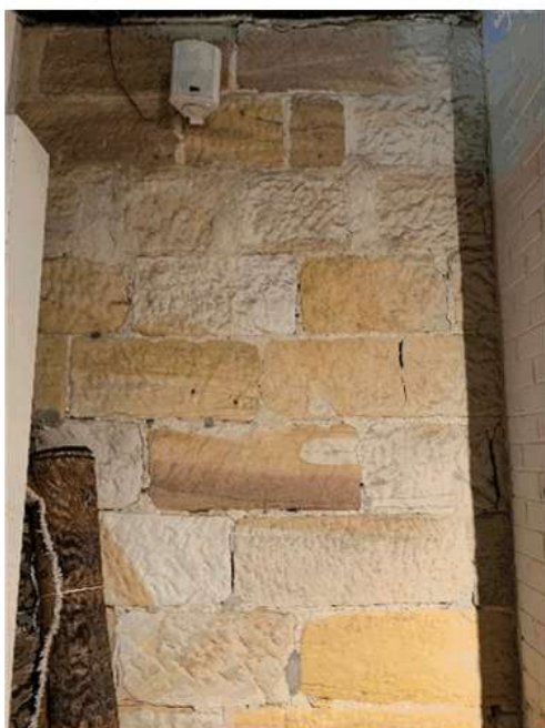
Figure 81: Basement level mass stone walling
