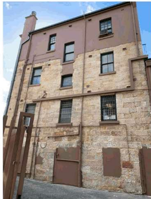
Figure 49: Rear elevation window openings showing the original window arrangements of the basement, ground and first floor level, with some openings retaining their 4 pane glazing arrangements despite the addition of security bars. Second floor level windows show the 9 + 1 glazing of the c.1909 scheme.
