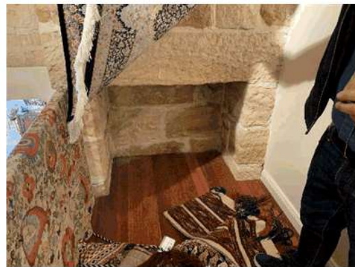
Figure 65: First floor level fireplace, with hearth covered by timber flooring
