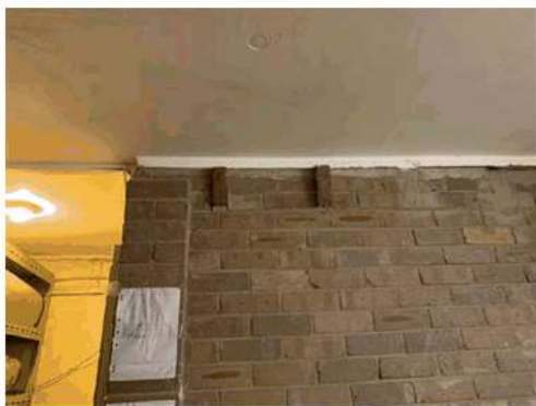
Figure 78: Basement level brick supporting walls
