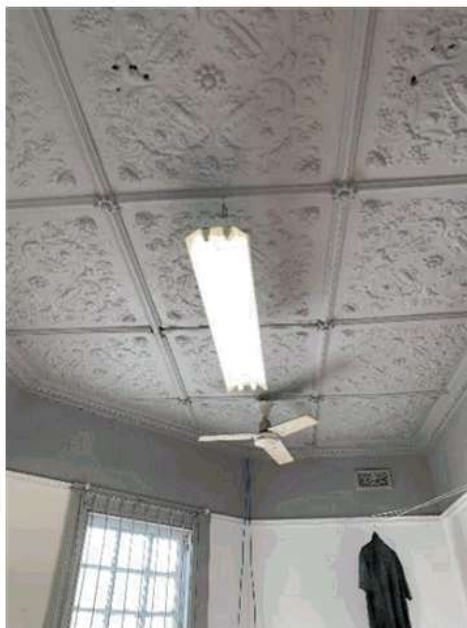
Figure 57: Level 2 decorative ceiling with waratah and flannel flower motifs. Accretion of modern fittings including fluorescent lighting and ceiling fans occur throughout.
