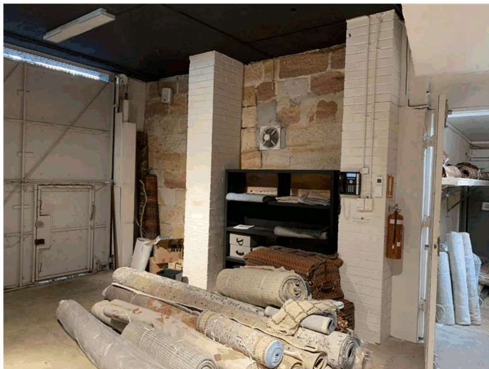
Figure 77: Basement level walls and support columns, mix of materials present, with services and intrusive exhaust fan element shown.
