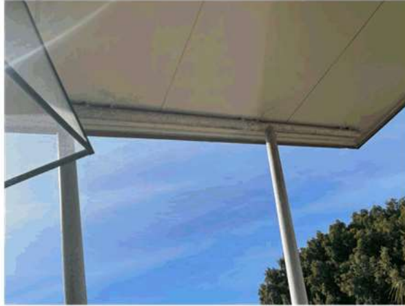
Figure 18. Connection of the steel V-shaped column to the soffit.
