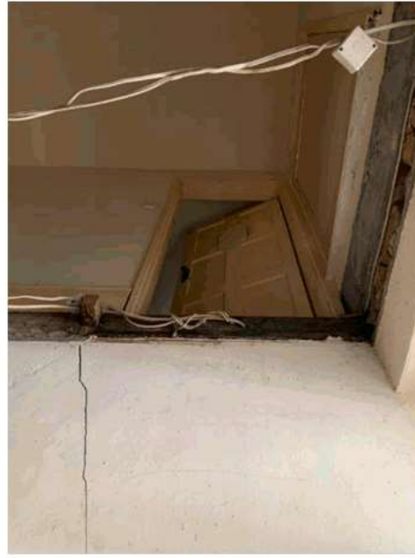
Figure 102: Interior, looking up at the first floor level, with crack plaster visible.
