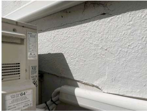
Figure 12. Northern exterior wall. The original form of tapered edge ground floor concrete slab, characteristic of Stossel's work, can still be seen— later infilled underneath as part of 1970s additions. (Source: Kieran McInerney, September 2021)
