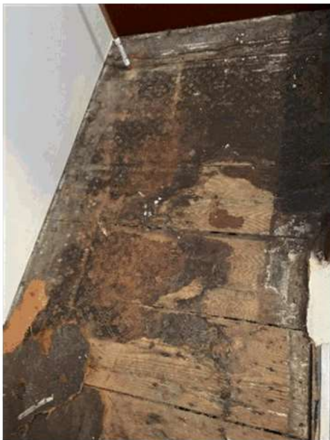
Figure 74: Multiple floor finishes visible on the southern stair landing
