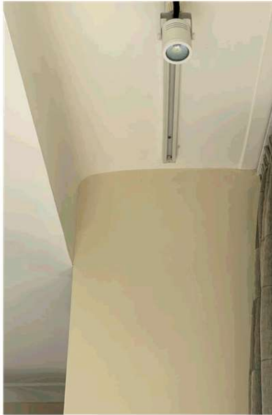
Figure 21. Ceiling cove, concealed pelmet, in living room which extends the width of front glass facade is typical of Stossel's work. This enables to the front facade to appear "glassier" and permits a thin edge to the roof soffit, achieving an even thickness frame around the first floor façade. It also hides the curtain mechanism with curtain fabric typically playing a key role in Stossel's interiors.
