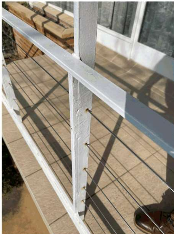
Figure 19. Detail of the steel balustrade which originally spanned the width of the front façade. Original mesh infill panels have been removed and replaced by stainless steel cable.
