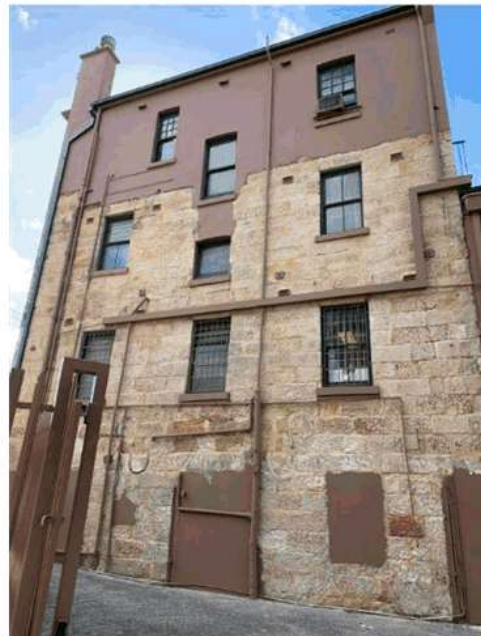
Figure 54: Rear elevation window openings showing the original window arrangements of the basement, ground and first floor level, with some openings retaining their 4 pane glazing arrangements despite the addition of security bars. Second floor level windows show the 9+1 glazing of the c.1909 scheme.
