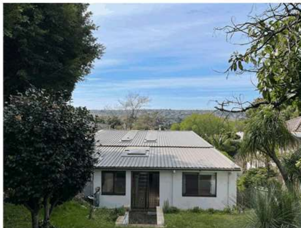
Figure 13. View from back garden showing aluminium windows of 1970s additions. The mono pitch, almost flat, skillion roof falls to the rear of the site. It has been extended back at the same fall as part of the 1977 additions.
