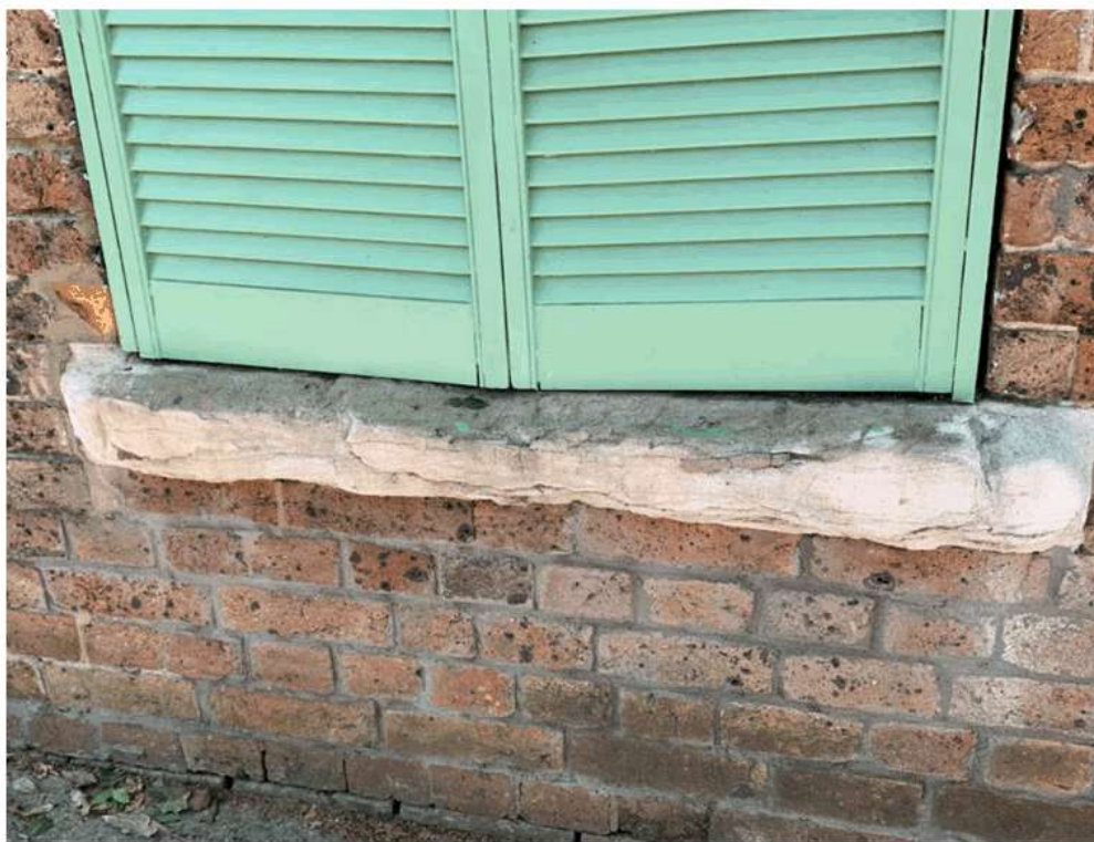
Figure 37: Weathered sandstone windowsill of 545 Glenmore Road, March 2020.
