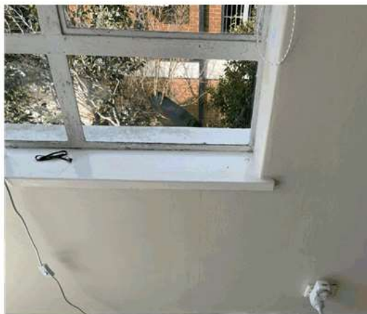
Figure 22. Typical window sill detail on original steel windows.
