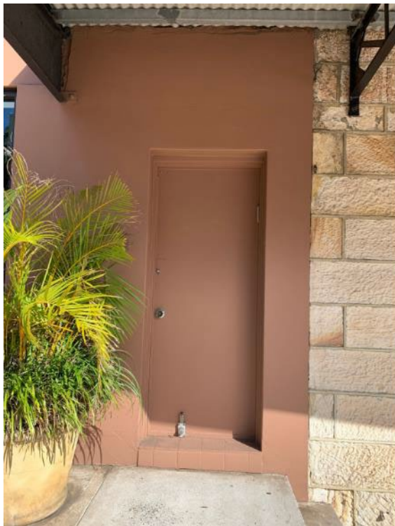
Figure 53: Door opening to 1980s showroom and transition from sandstone to modern fabric, New South Head Road elevation.
