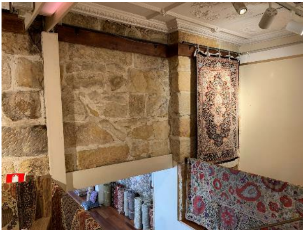
Figure 69: First floor level exposed sandstone walls, with gallery rug display rails affixed to the top part of the wall
