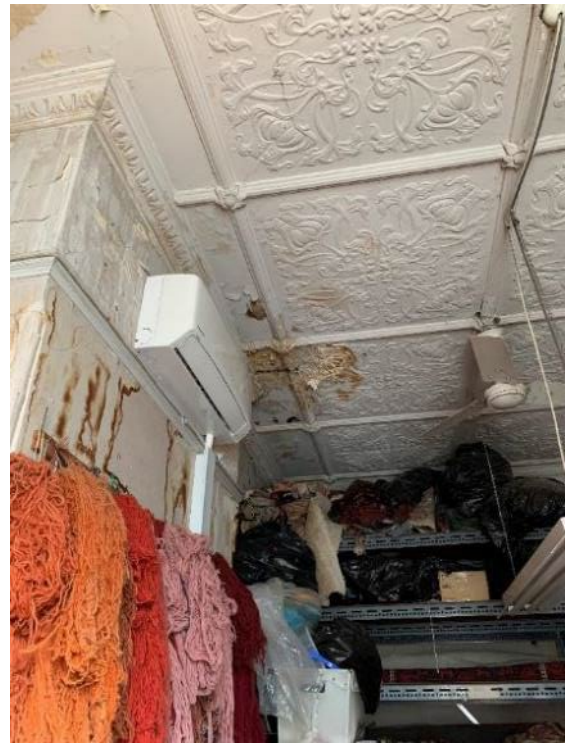
Figure 61: Decorative ceiling on Level 2. Prior water damage to the ceiling is evident in this space.
