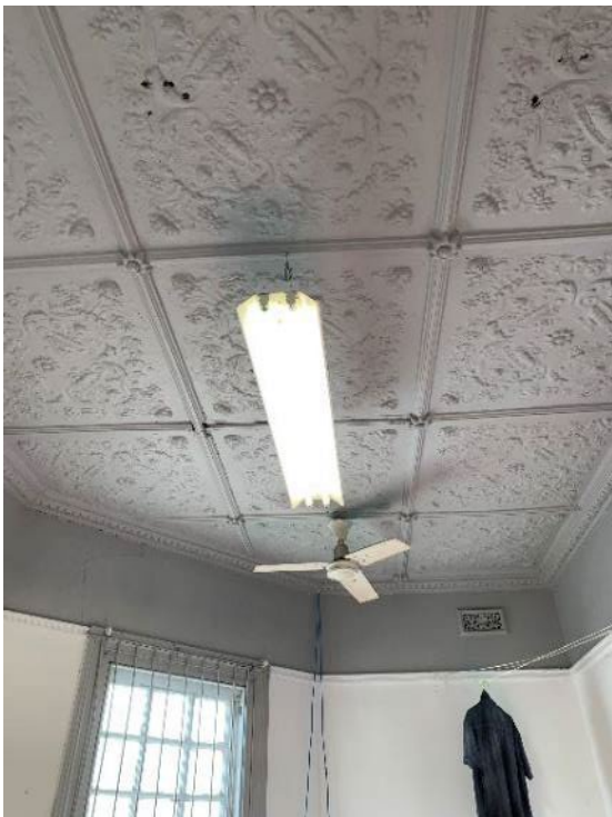
Figure 62: Level 2 decorative ceiling with waratah and flannel flower motifs. Accretion of modern fittings including fluorescent lighting and ceiling fans occur throughout.
