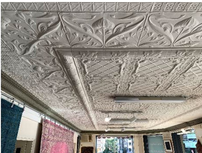
Figure 71: Pressed metal ceiling at ground floor level to the principal showroom space, formerly the main bar.
