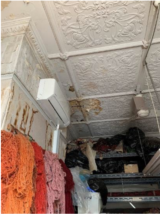
Figure 64: Level 2 decorative ceiling and cornice elements, with water damage visible
