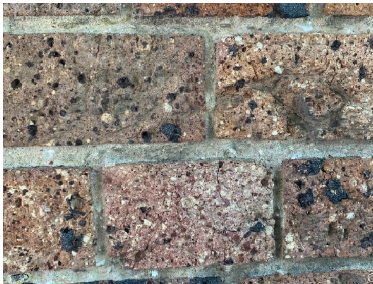
Figure 36: Shell pozzolans visible in the mortar of 549 Glenmore Road
