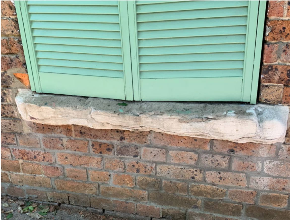
Figure 37: Weathered sandstone windowsill of 545 Glenmore Road, March 2020.
