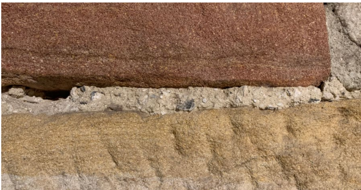
Figure 87: Detail of existing mortar in the sandstone walling, with shell pozzolans visible
