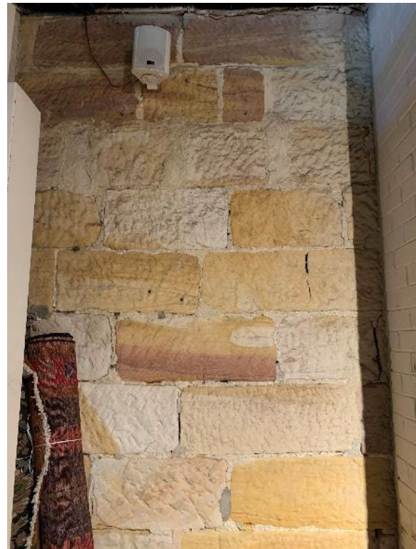
Figure 86: Basement level mass stone walling
