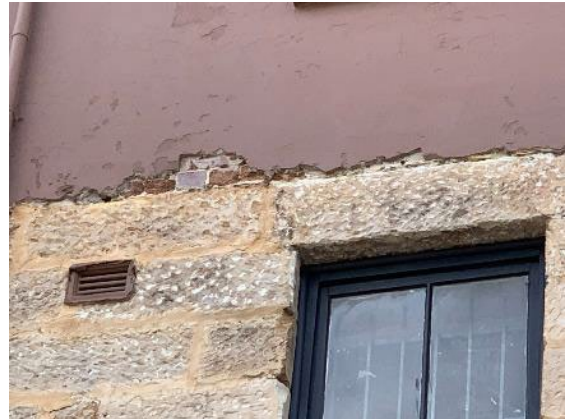
Figure 56: Detail of the change in construction material and finishes between first floor and second floor levels
