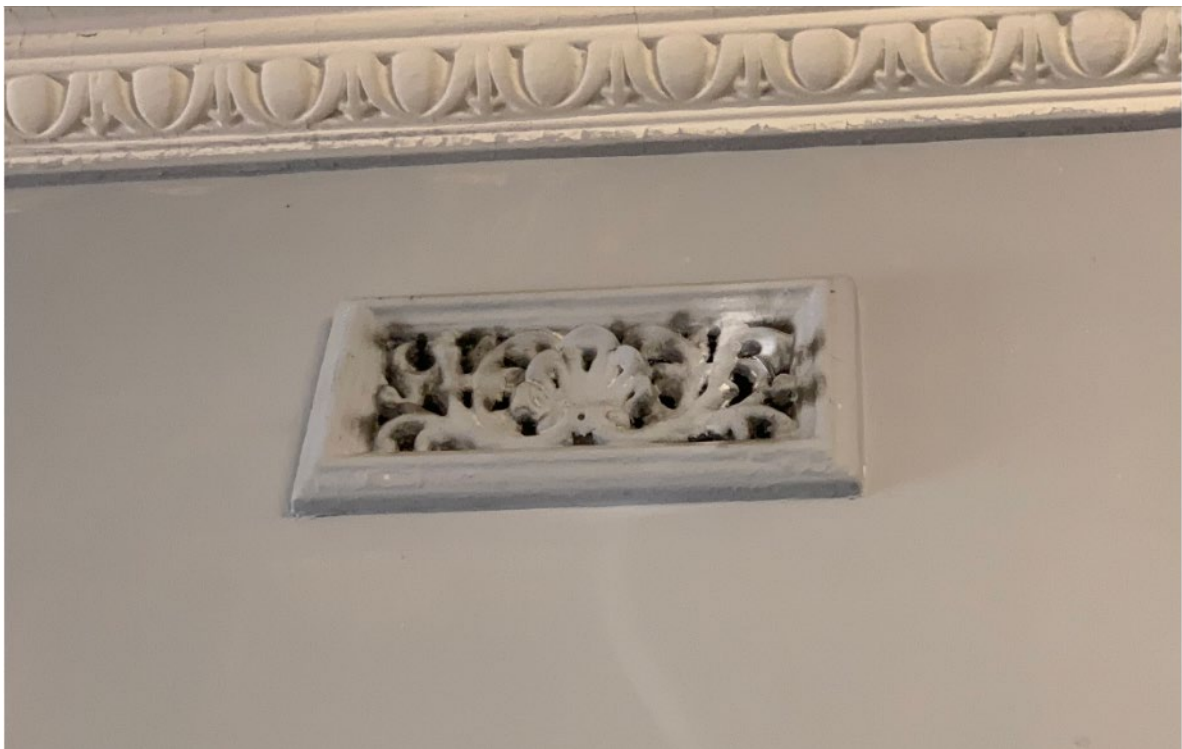
Figure 66: Level 2 feathered room vent and egg and dart cornice.
