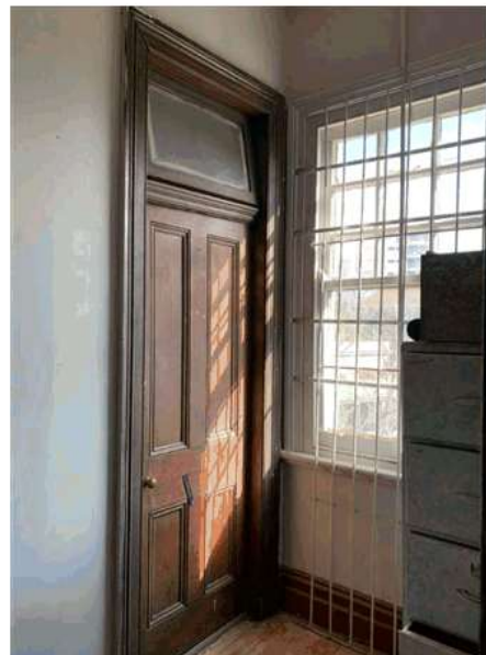
Figure 60: Level 2 c.1909 door, with fanlight and joinery with original window also visible
