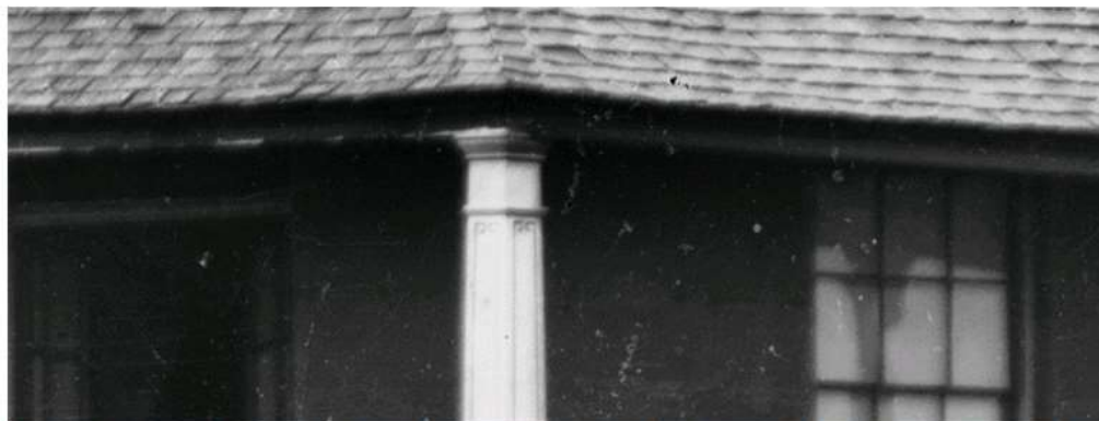
Figure 83: Magnified detail of the first floor level singled balcony support post from Nicholson's Hotel on the south-eastern corner of New South Head Road & Glenmore Roads, Rushcutters Bay (with adjacent Billiard Bagatele Room and William Harris's produce store). c1870-1875 (Source: American & Australasian Photographic Company via Mitchell Library, SLNSW https://archival.sl.nsw.gov.au/Details/archive/110040845 )
