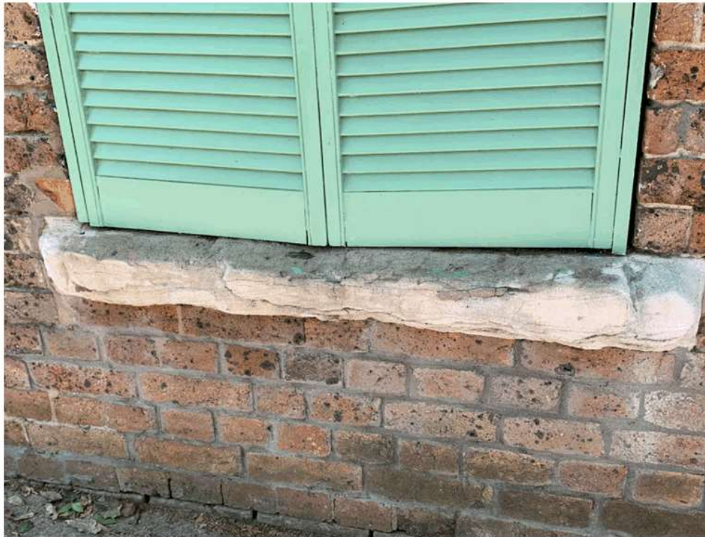
Figure 39: Weathered sandstone windowsill of 545 Glenmore Road, March 2020.
