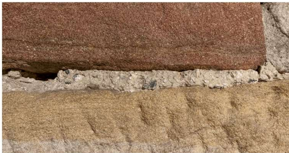
Figure 82: Detail of existing mortar in the sandstone walling, with shell pozzolans visible
