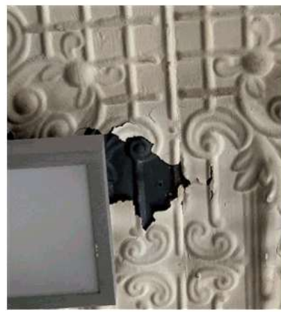
Figure 67: Pressed metal ceiling detail at ground floor level to the principal showroom space, formerly the main bar.
