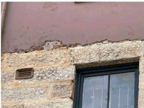
Figure 51: Detail of the change in construction material and finishes between first floor and second floor levels
