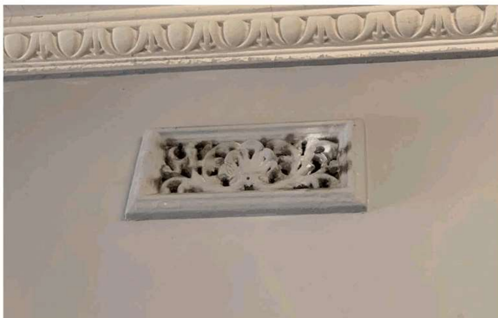
Figure 61: Level 2 feathered room vent and egg and dart cornice.
