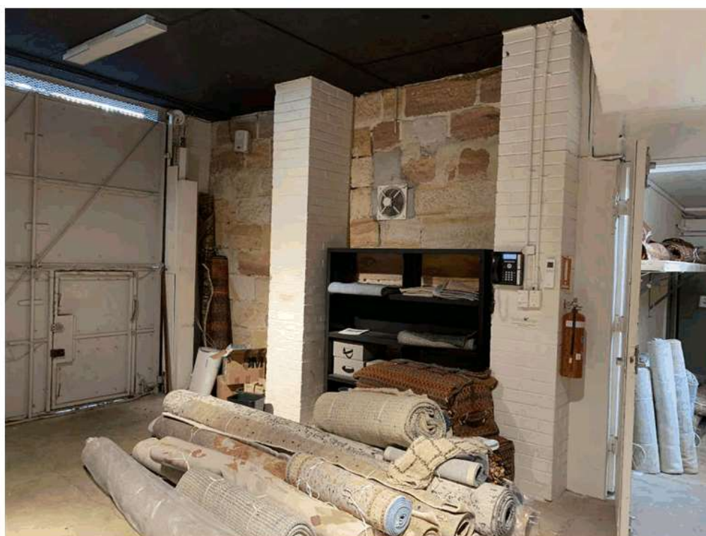
Figure 77: Basement level walls and support columns, mix of materials present, with services and intrusive exhaust fan element shown.
