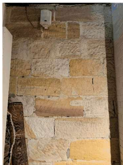
Figure 81: Basement level mass stone walling
