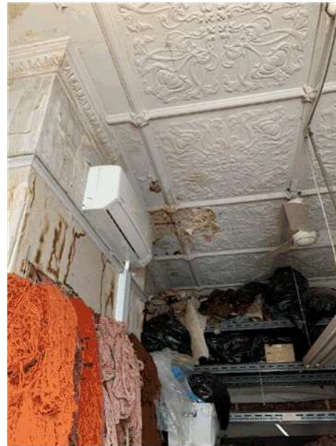
Figure 56: Decorative ceiling on Level 2. Prior water damage to the ceiling is evident in this space.
