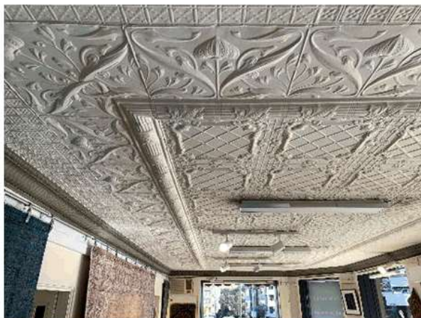
Figure 66: Pressed metal ceiling at ground floor level to the principal showroom space, formerly the main bar.
