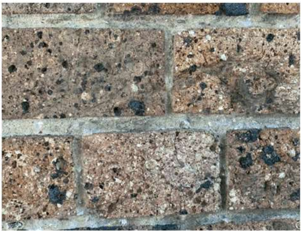
Figure 38: Shell pozzolans visible in the mortar of 549 Glenmore Road
