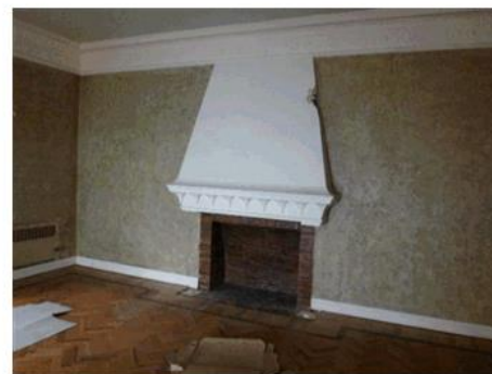
Figure 70: Fireplace as at 24 January 2020, with columns removed and minor damage to the hood.
