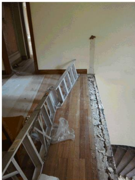
Figure 87: Balustrade to the first floor level landing has been removed
