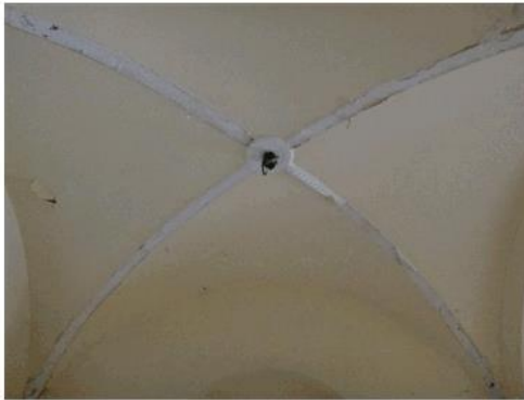
Figure 73: Vaulted ceiling to entryway. Evidence of decoration to ribs of the vaulted ceiling having been removed.
