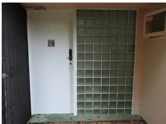
Figure 7.17: Front door with glass block sidelight. (Source: Robertson & Hindmarsh Pty Ltd, 1 March 2022)
