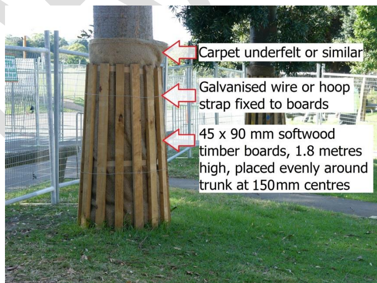
Figure 7 – Detail of Trunk Protection
