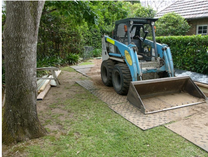
Figure 8 – Showing typical detail for truck mats.
