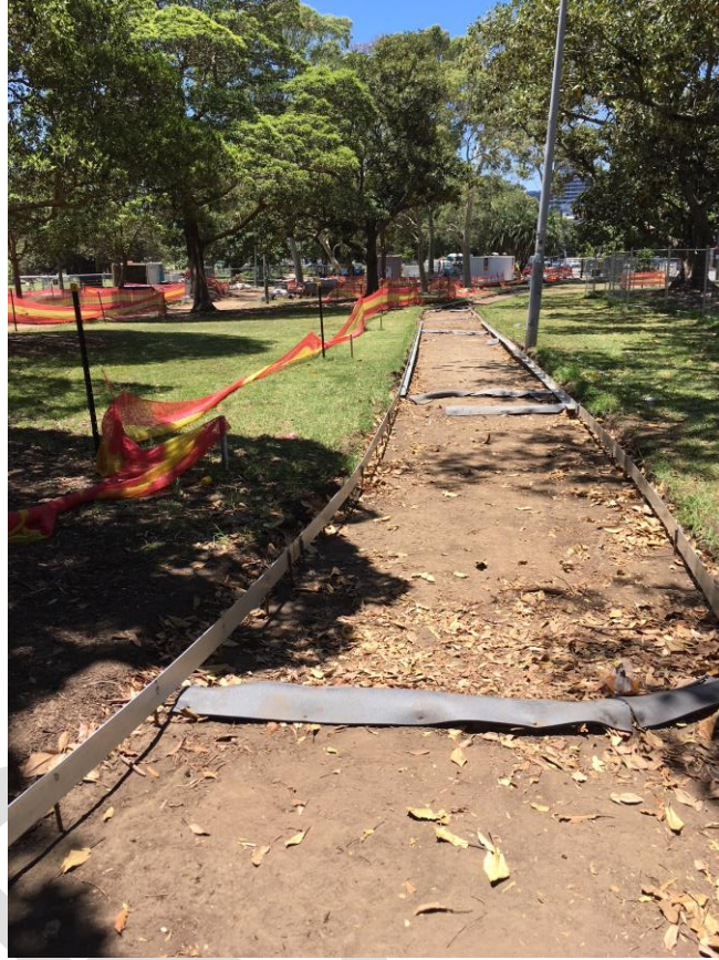
Figure 3 – Woody roots retained in the path sub-grade and protected prior to placement of sub-base material with Xcellon Expansion Joint Foam (Victoria Park, Sydney).
