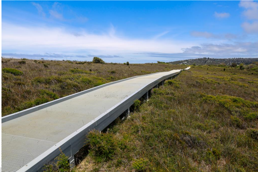
Figure 4 – Low boardwalk constructed using PermaStruct® RapidDeck
