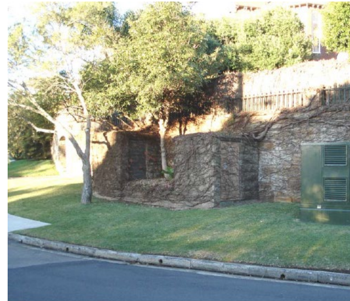
Figure 14: Gilliver Avenue underground vault type substation (2012) set into sandstone walling. (Source: Pennington, 2012 p.635)
