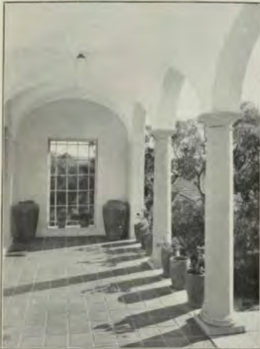
The entrance of this house is of stone, the walls were stained. The plastered ceiling is designed to be suitably painted later on and the paving is of large, red, French quarry tiles. Through the handsome grilled opening at the end an uninterrupted view over the trees in Bellevue Hill is obtained.
