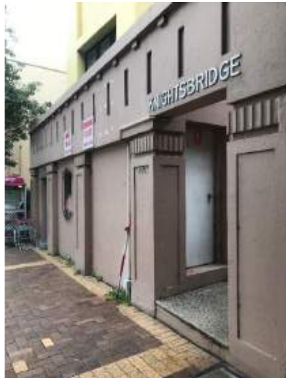
Figure 28 – Masonry wall and lower ground floor amenities area separates main building structure from street.
