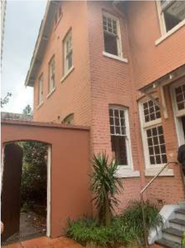
Figure 55 – Western elevation with later addition painted brickwork.
