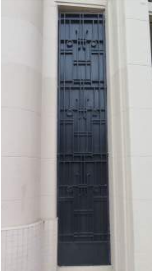
Figure 14 - Original decorative metal grille over window
