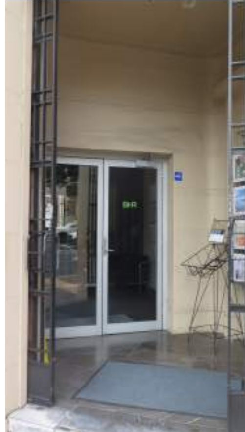
Figure 15 – Corner entry porch with decorative sliding grille and later addition door opening with aluminium doors
