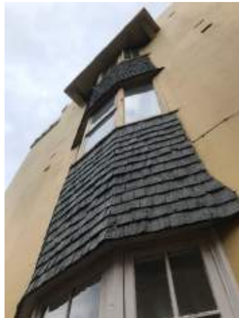
Figure 32 – Detail of bay windows clad with timber shingles expressing the feature bay.
