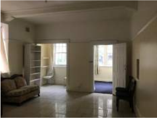
Figure 33 – Interior fabric, ground floor apartment with plaster finish masonry walls, timber architraves, skirting and pictures rails.
