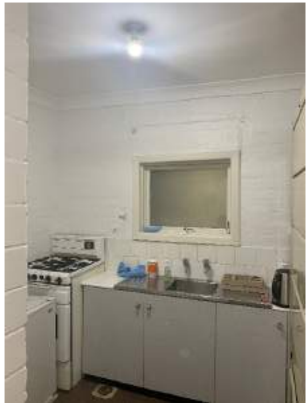
Figure 126 – Kitchen within secondary tenancy at northern wing of ground-floor. Painted face brickwork walls.
