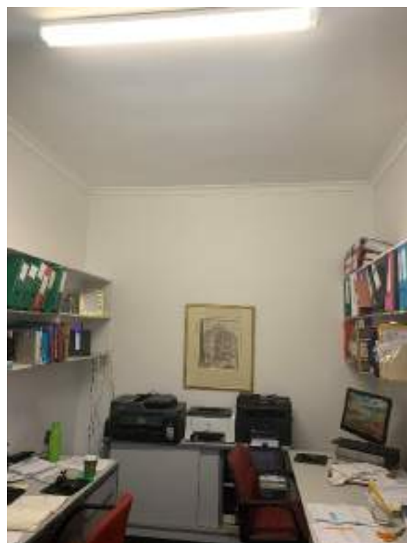
Figure 124 – Office space within second tenancy at northern wing of ground floor. Later addition plasterboard ceiling and cornices.
