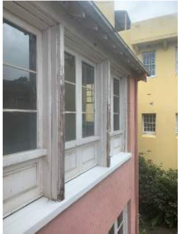
Figure 56 – Detail of eaves overhang and exposed timber rafters to roof at rear of dwelling. Later addition windows.
