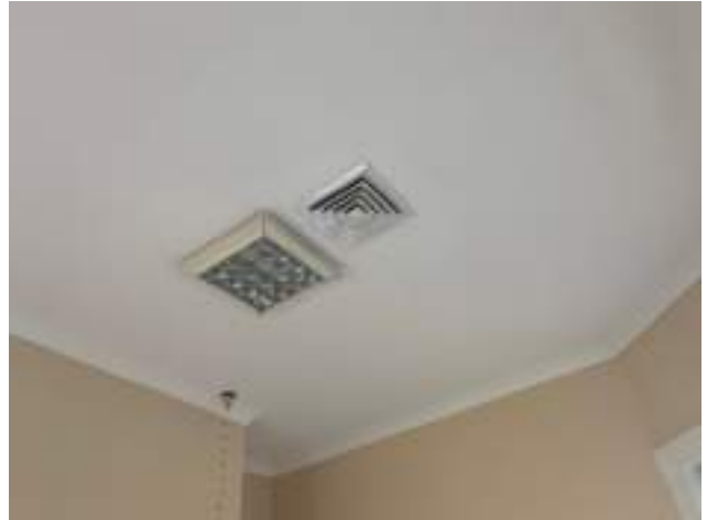
Figure 77 – First floor, south-western room with later addition, plasterboard ceiling and cornice and air condition vent.
