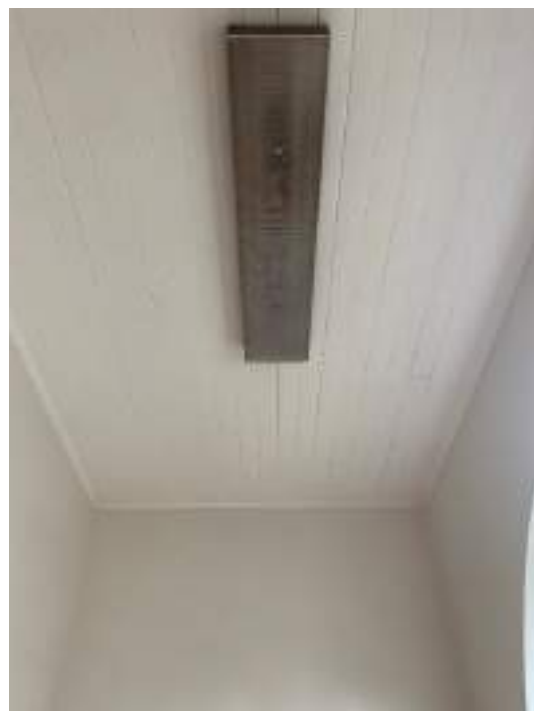
Figure 116 – Timber tongue-and-groove ceiling in enclosed veranda space.
