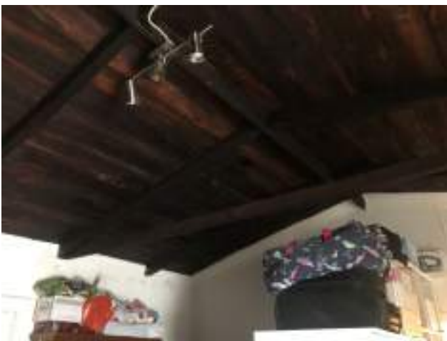
Figure 47 – Roof top apartment - timber roof structure with exposed stained beams and lining.
