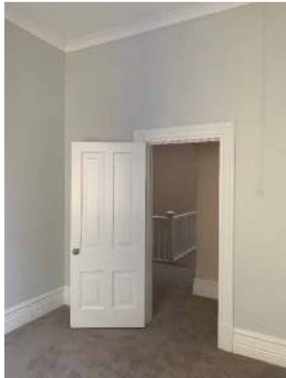
Figure 79 – First floor, later addition timber door with original timber architrave and skirting board.
