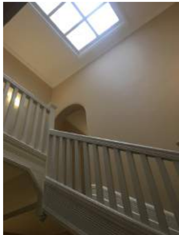
Figure 71 – Detail of timber balustrade to stair and timber framed skylight in ceiling.
