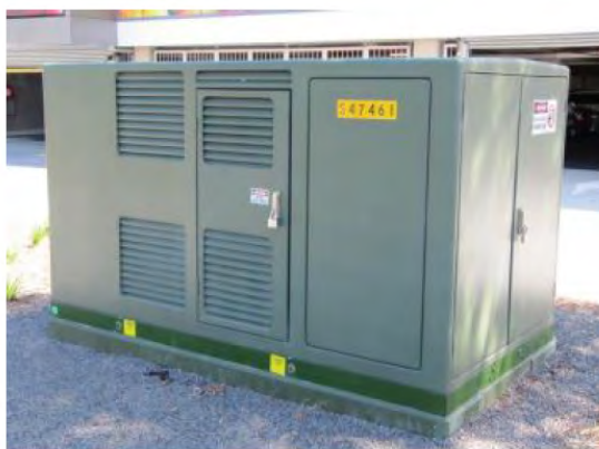
Figure 1: Kiosk substation: address unknown Source: Ausgrid
