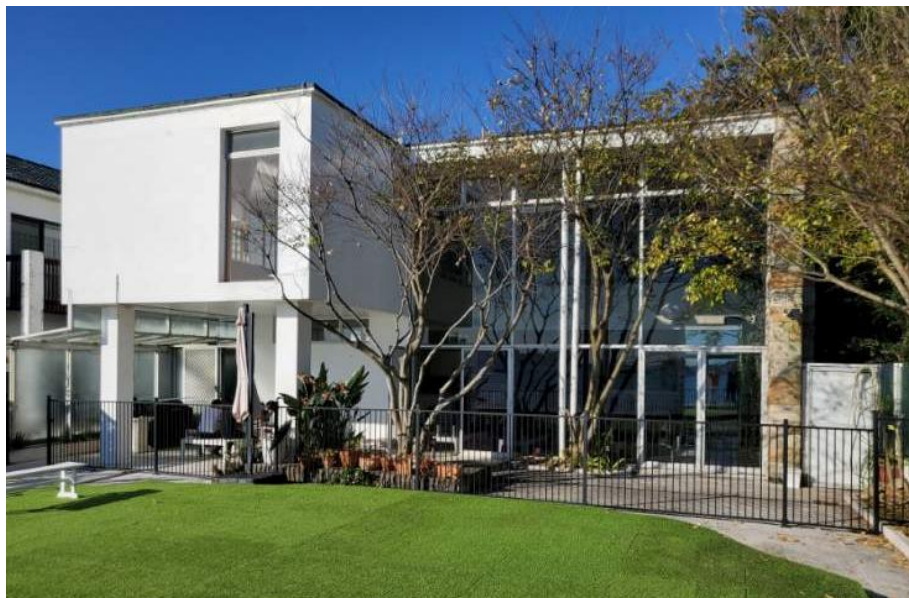
28 Western elevation of the Lapin House. The square piers supporting the cantilevered section of the first floor may encase the original steel pipe columns, which have been retained in front of the Living Room glazing. Original doors and louvres have been replaced
