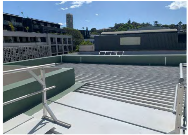
Figure 11 View to the roofspace comprising a contemporary corrugated metal sheeting material.
