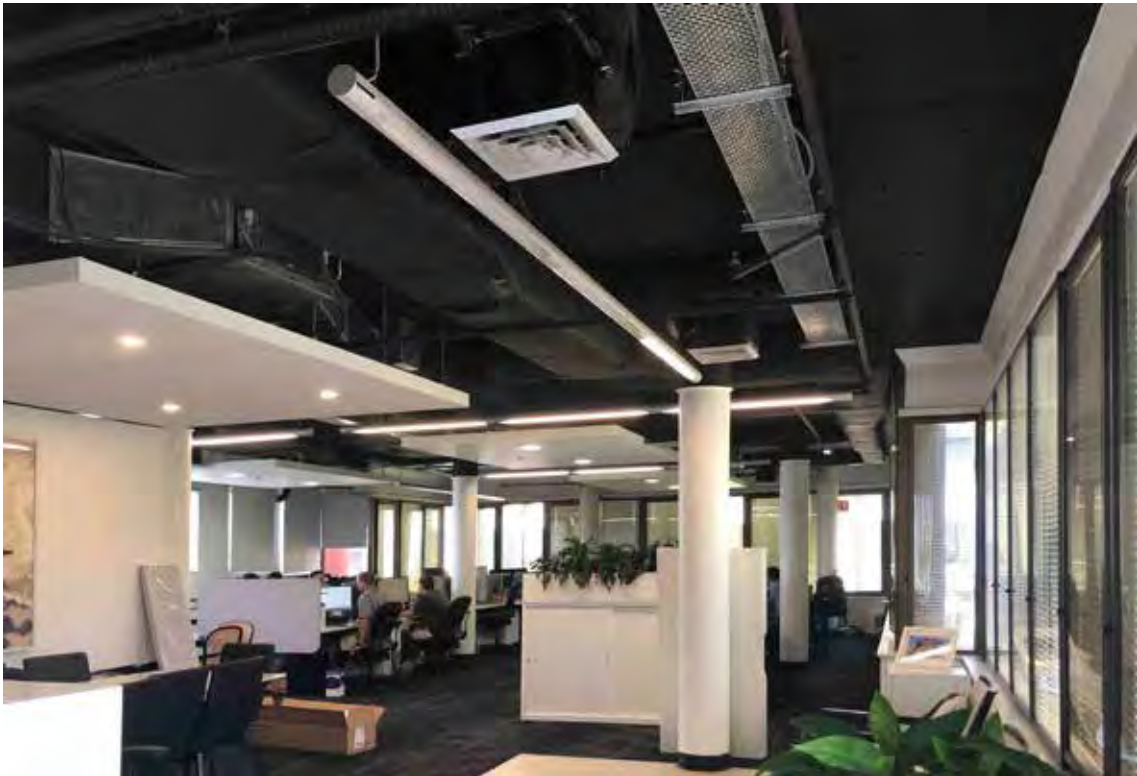
Figure 49 | Office spaces on the top floor (Level 3). Contemporary standard office fit-out. The ceiling is the concrete slab soffit with exposed services. Again, the coffering was never built.
