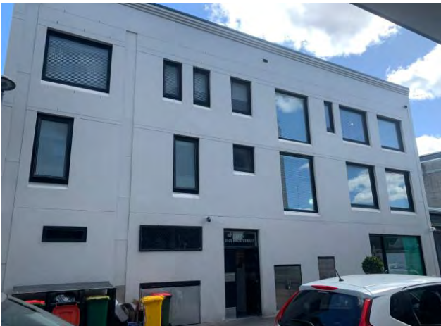
Figure 10 View to the rear (north) elevation from Knox Lane. This elevation has been rendered and comprises contemporary aluminium-framed windows.
