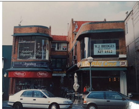
Figure 7: This photograph of Nos. 21-15 Knox Street in the 1980s recorded the original features of the building as designed by Evans in 1955 inclusive of the steel framed windows and face brick walls to Knox Street.
