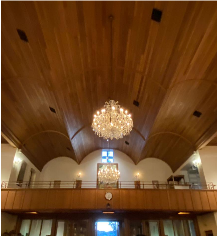
Figure 10. Internal, view of triple-vaulted panelled ceiling and rear balcony. (Source: Woollahra Council, 2023)
