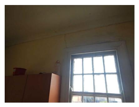
**Photograph 17.** Cracked interior skin of exterior masonry wall. Potentially due to lintel corrosion.
