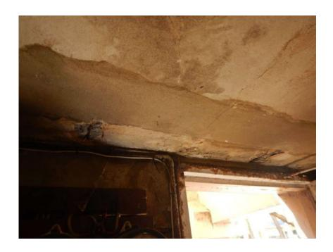
**Photograph 6.** Concrete ceiling and roof slab to the street level Flat. Note the spalling and deterioration of the slab due to moisture ingress from above.
