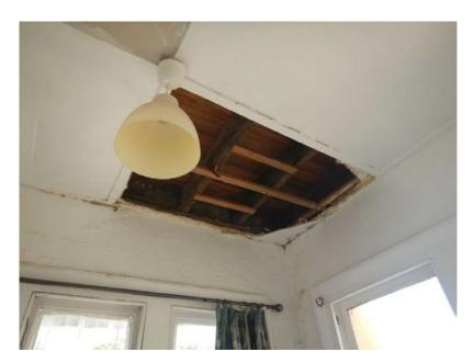
**Photograph 12.** Ceiling showing timber floor construction. Note the timber wall plate founding on the inner skin of masonry. The masonry exhibits signs of moisture ingress with blistering paint. Isolation between the timber wall plate and the masonry is not known.
