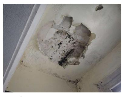
**Photograph 16.** Ceiling/ roof slab corroded reinforcement where building line steps back.
