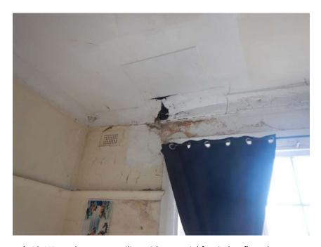
**Photograph 18.** Water damage to ceiling with potential for timber floor dry rot.
