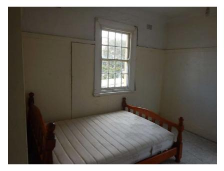
**Photograph 19.** Extensive addition of cover boarding to the interior face of the exterior wall due to water ingress through the wall.
