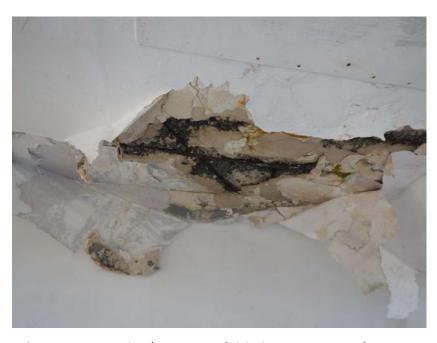
**Photograph 14.** Concrete ceiling/ exterior roof slab showing sever reinforcement corrosion, concrete cancer.
