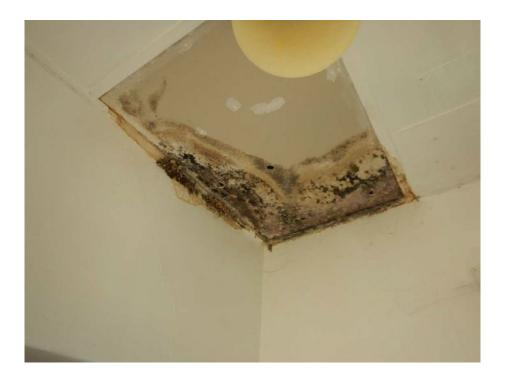
**Photograph 13**. Ceiling located below a bathroom showing water damage and potential effect on timber floor framing due to dry rot.
