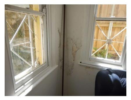
**Photograph 9.** Ground floor unit at the Norther Eastern corner. Note the moisture ingress to the inside face of the wall. Structurally relates to the potential effect on timber floor joists supported by the wall.
