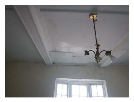
**Photograph 15.** Ceiling access covers against the East Exterior Wall due to water ingress. Effect on the timber floor joists which would span between the perpendicular main beams is unknown.
