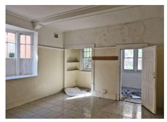
**Figure 3.6**Photograph of a flat in 138-140 New South Head Road. Note the pronounced mould on the upper wall, and the collapsed ceiling sections on the floor, caused by water ingress
