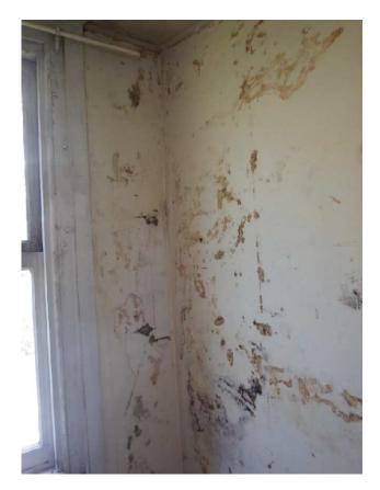
**Photograph 12.** Internal masonry wall showing moisture effects and potential effect on the timber floor.
