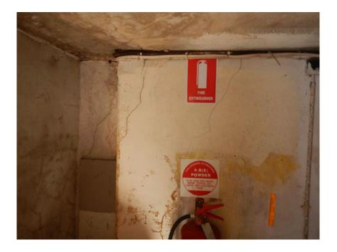
**Photograph 7.** Electrical meter room at Ground Level Street side. Note the cracked masonry walls and water-stained ceiling / roof slab.
