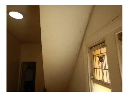
**Photograph 10.** Soffit of reinforced concrete stair flight with hair line longitudinally parallel to exterior wall indicative of reinforcement corrosion.
