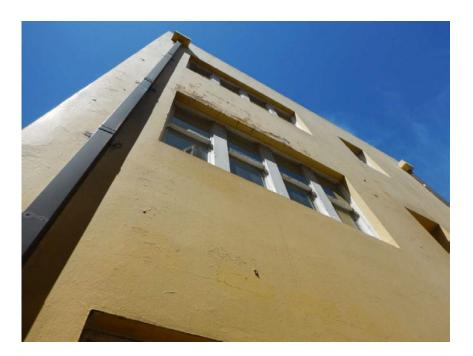
**Photograph 5.** Northern Facade. Note the spalling of the window head lintel.
