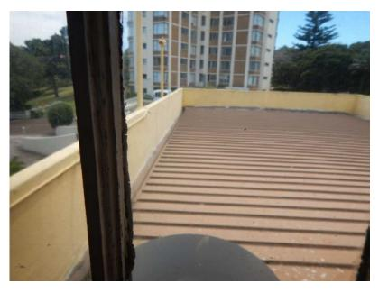
**Photograph 22.** Roof over the Northern area of the building, metal deck with shallow side falls to the East and West. Note the laterally unrestrained parapet walls. Note the shallow and narrow gutters.
