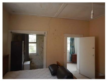
**Photograph 11.** Cracked internal masonry load bearing wall.
