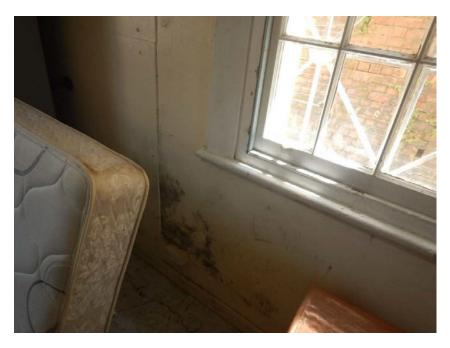
**Photograph 8.** Ground floor Flat. North side. Note the water damage to the interior masonry wall and potential effect on timber floor framing in contact with the wall. Also note the application of a cover applied to the inside face of the wall.
