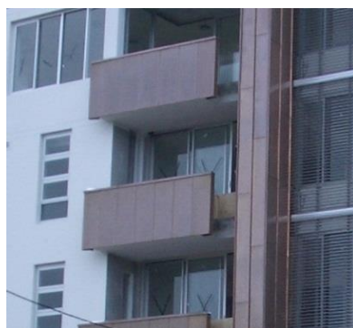
FIGURE 3 Part projecting balcony
