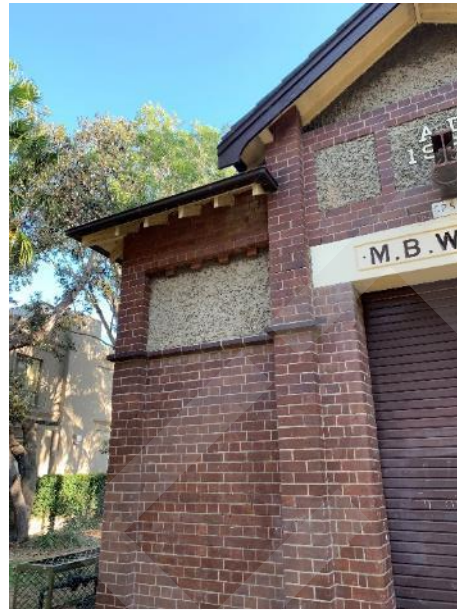
Figure 85: View of minor cracking in brick work from metal beam in the sewage pumping station
