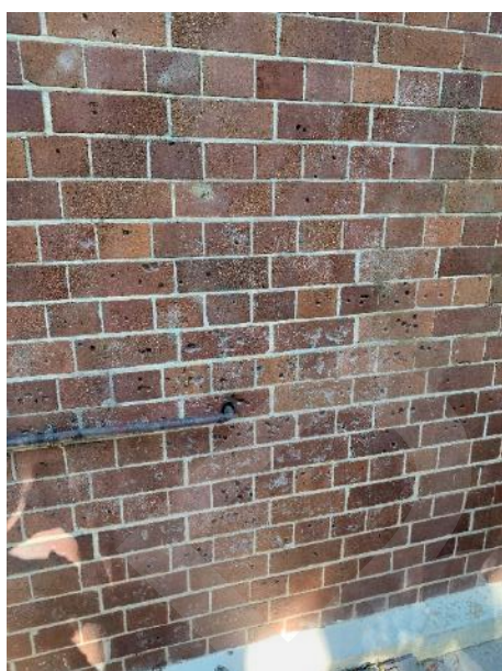
Figure 82: View of damage to brick work from opening of access pit on the side of the sewage pumping station
