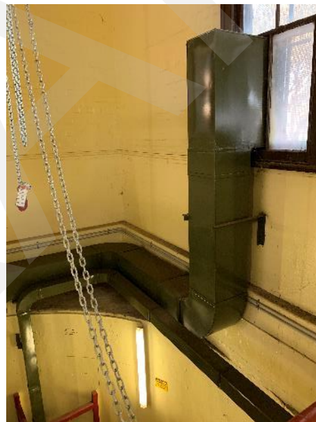
Figure 50: View of the internal ventilation flue of the sewage pumping station
