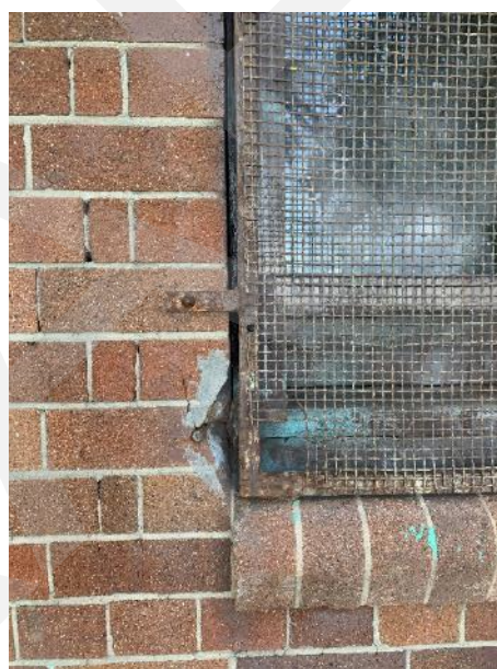
Figure 83: View of damage to brick work from metal bolts on the side of the sewage pumping station
