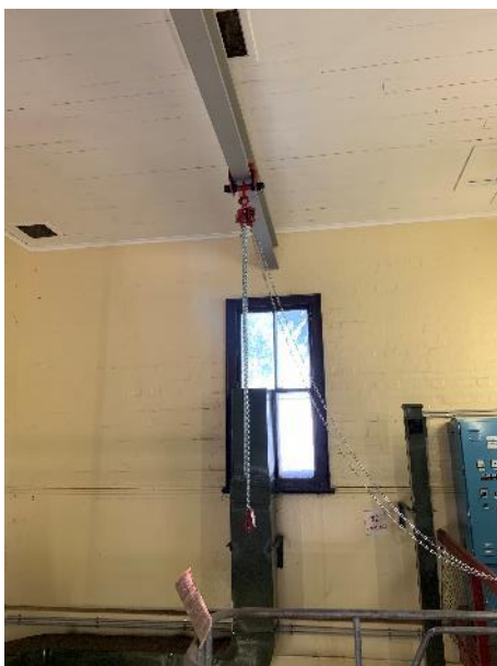
Figure 55: View of the internal crane in the sewage pumping station
