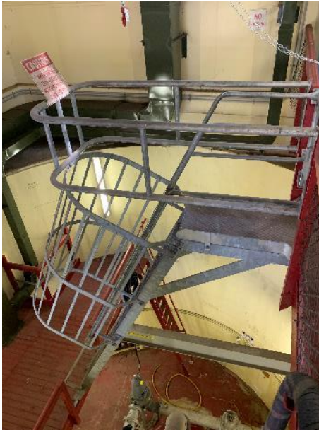
Figure 35: View of the internal access ladder and pumping equipment of the sewage pumping station
