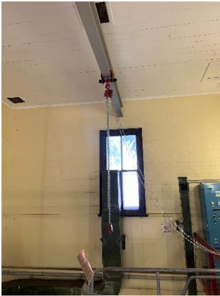
Figure 47: View of the internal crane in the sewage pumping station
