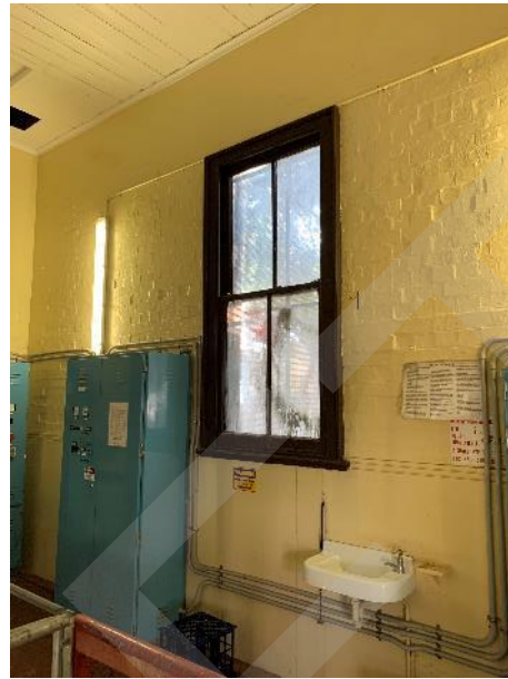
Figure 48: View of the timber framed double hung sash window of the sewage pumping station
