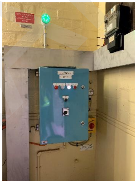
Figure 42: View of the electrical switchboard of the sewage pumping station
