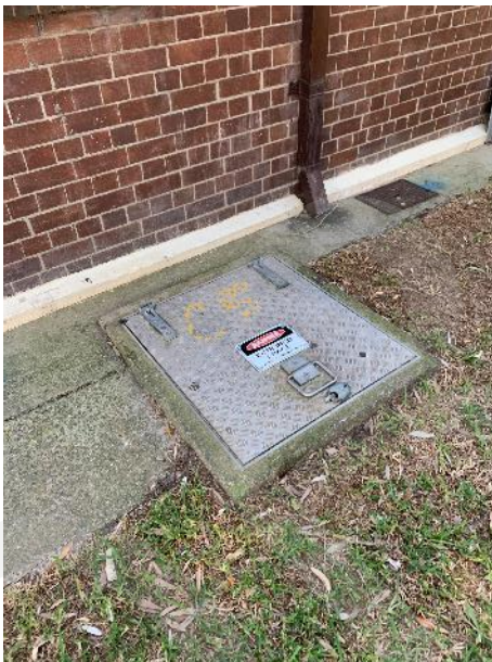
Figure 30: View of the modern access pits of the sewage pumping station
