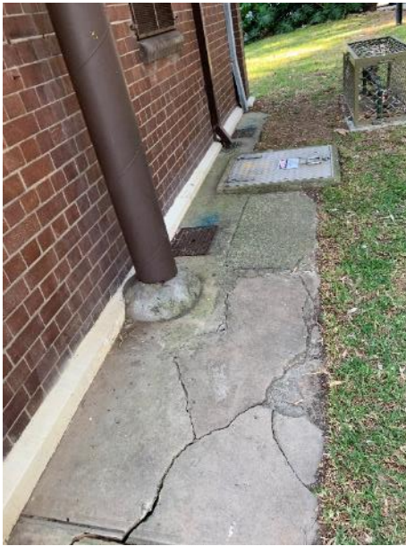
Figure 84: View of damage to concrete path around the sewage pumping station
