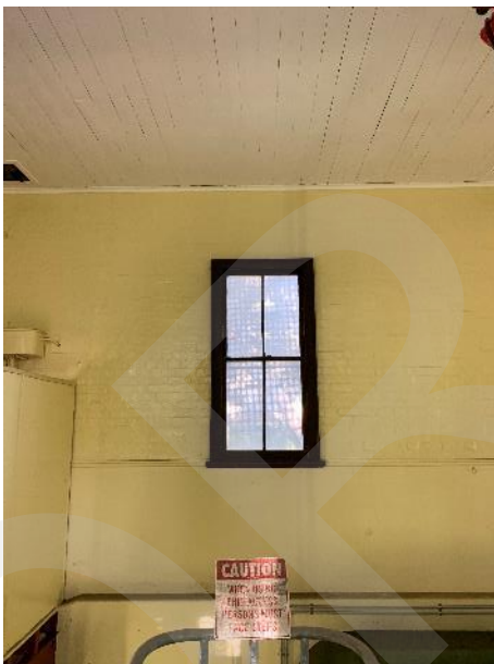
Figure 49: View of the timber framed double hung sash window of the sewage pumping station
