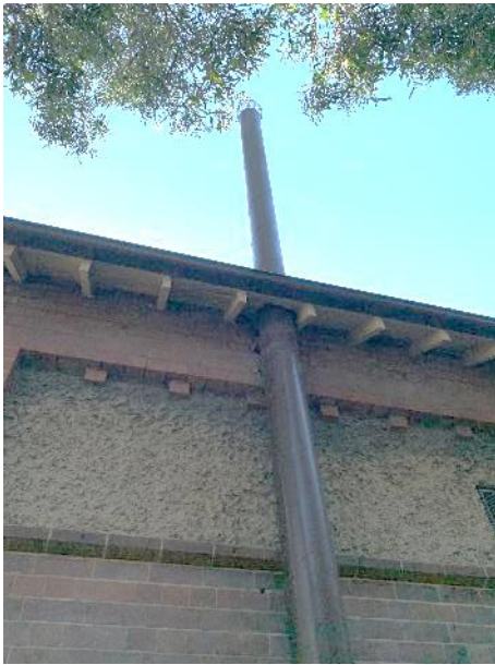
Figure 28: View of the vent of the sewage pumping station
