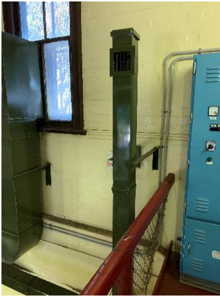
Figure 51: View of the internal ventilation flue of the sewage pumping station
