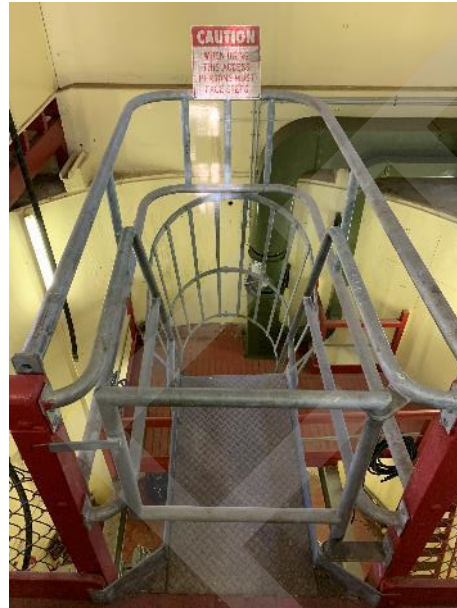
Figure 36: View of the internal access ladder and pumping equipment of the sewage pumping station
