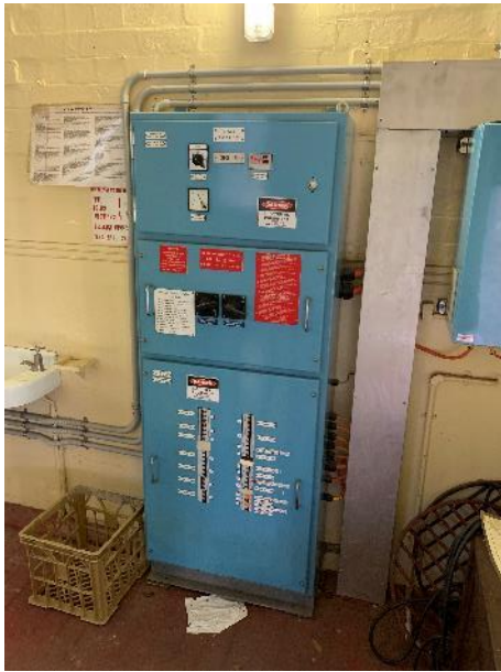
Figure 43: View of the electrical switchboard of the sewage pumping station
