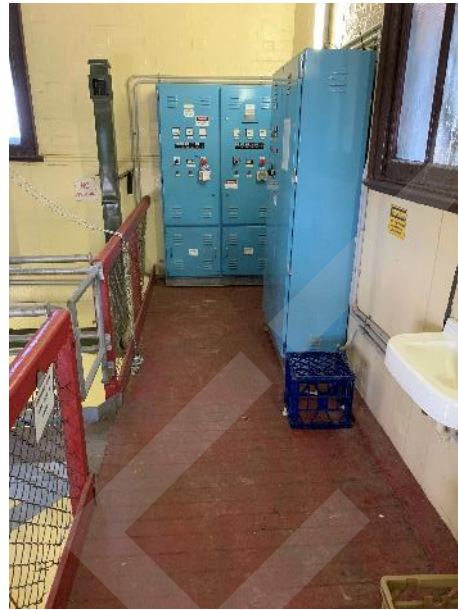
Figure 44: View of the electrical switchboard of the sewage pumping station
