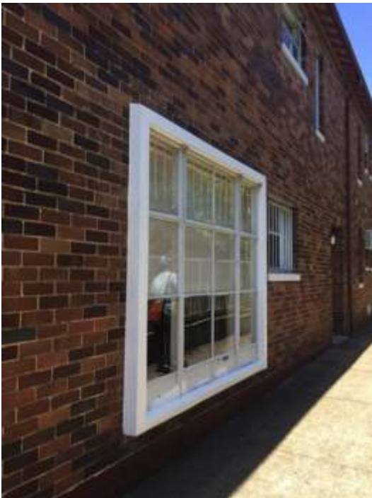
Figure 21. Extensive steel framed glazing to dining space of apartment 5 with cement rendered framed window surround. (Author photo)
