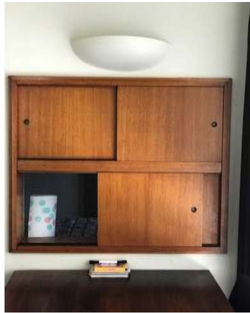
Figure 35. The maisonette (apartment 5) has a light coloured timber veneer sliding door servery unit between the kitchen and the dining nook. (Author photo)
