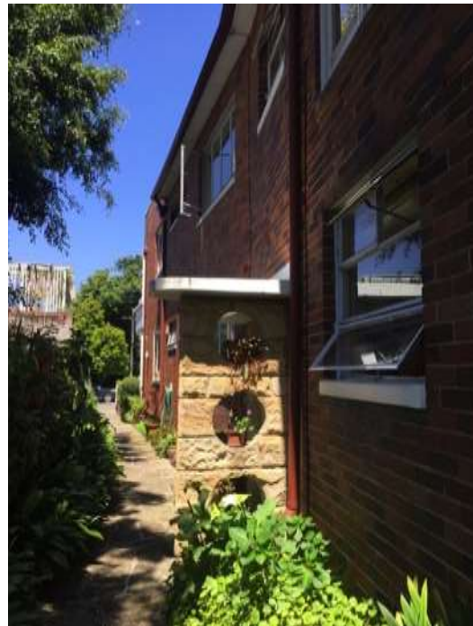
Figure 22. Curved concrete slab awning and ashlar sandstone blade wall punctuated by 3 circular openings at the lobby entry. (Author photo)
