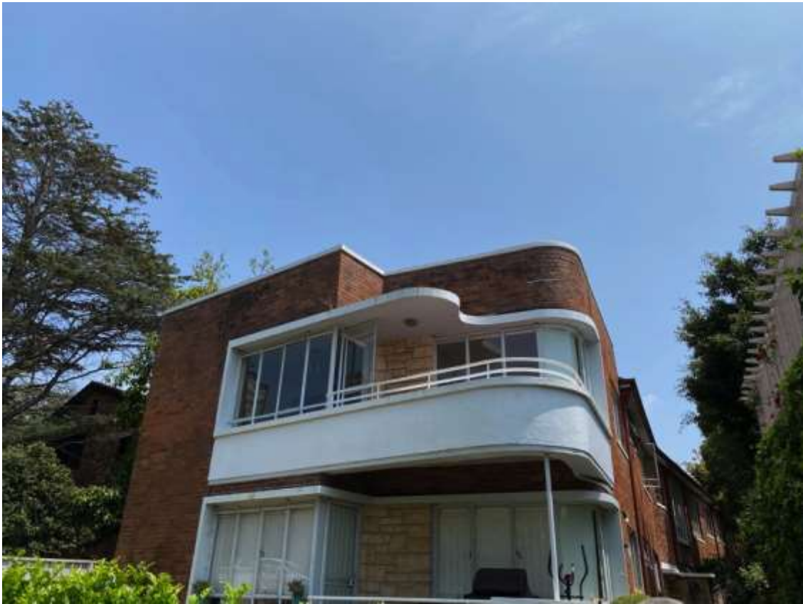
Figure 25. Trelawney Street façade detail: Note distinctive “S” shaped first floor concrete awning slab edge, curved sandstone feature panels and bulkhead light. (Source: Author photo)
