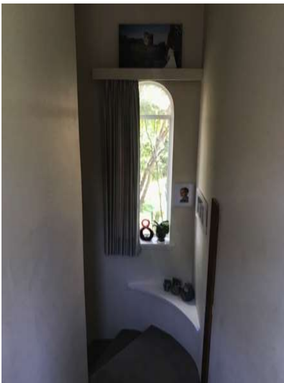
Figure 28. Tall steel framed glazing to maisonette stair with semi-circular operable window at head. (Author photo)
