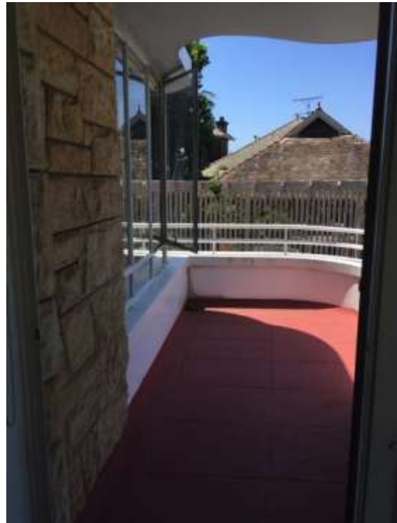
Figure 24. Curved concrete slab awning and curved and angular dressed ashlar sandstone wall with slender steel framed windows and curved handrails to front facade. (Author photo)
