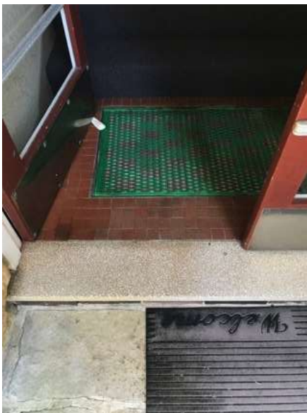
Figure 32. The entry lobby has an entry landing of 2 inch x 2 inch unglazed terracotta tiles and a threshold sill of honey coloured terrazzo. (Author photo)
