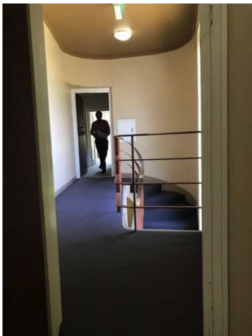
Figure 38. The main stair has curved winders and a curved balustrade of welded steel flats typical of cinema buildings of the 1930s. Ceilings are also curved. Blukhead light matches extrnal lights on street facade awning (Author photo)
