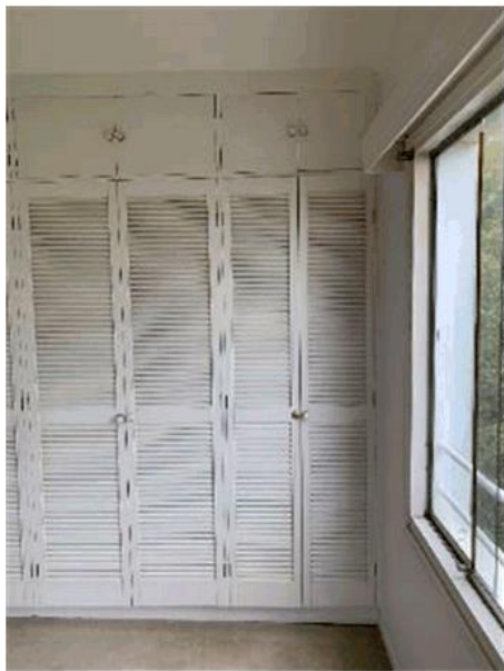
Figure 67: Built-in cabinetry in the former sleepout. The slight angle of the floor and flashing indicates the former exposed nature of the space.
