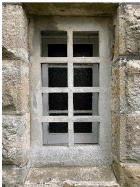
Figure 31: View of original concrete grille to the lower level store/laundry.
