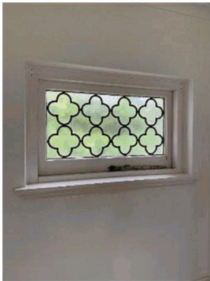
Figure 62: Moorish motif leadlight hopper window above the dressing table.
