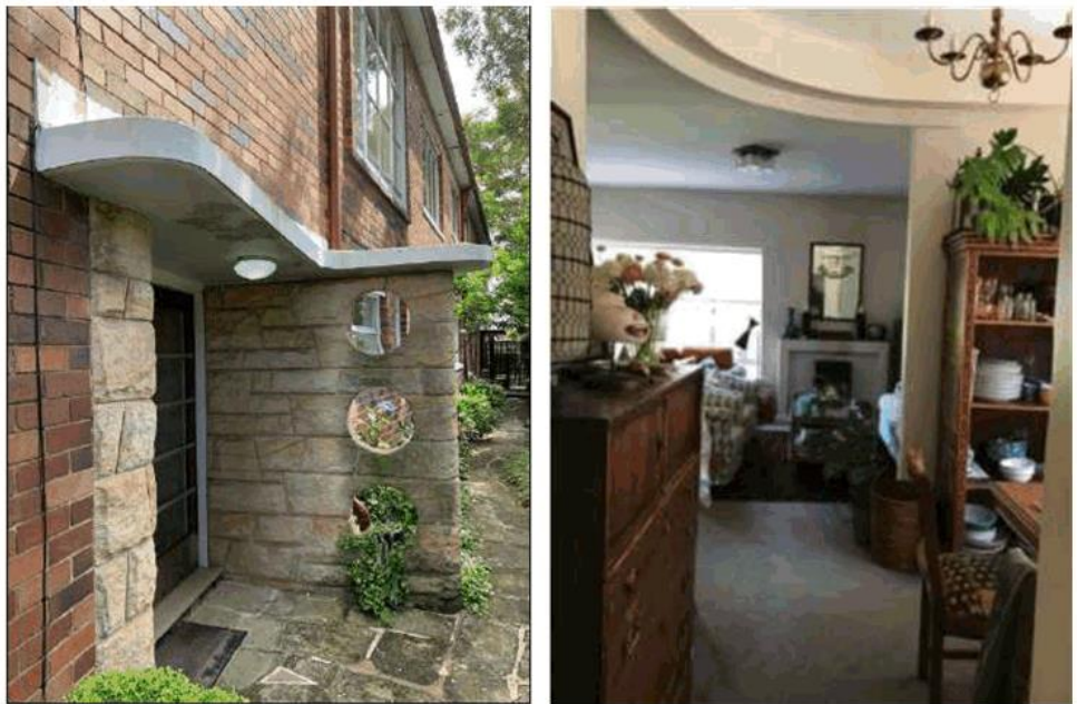
Figure 4 and 5: Main entry door with a curve concrete slab awning over an ashlar sandstone blade wall and curved 'streamlined' plasterwork.
