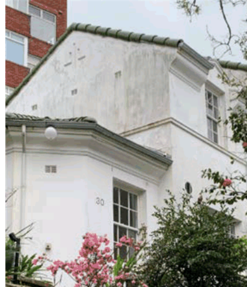
Figure 34: Staining and biological growth on the external wall
