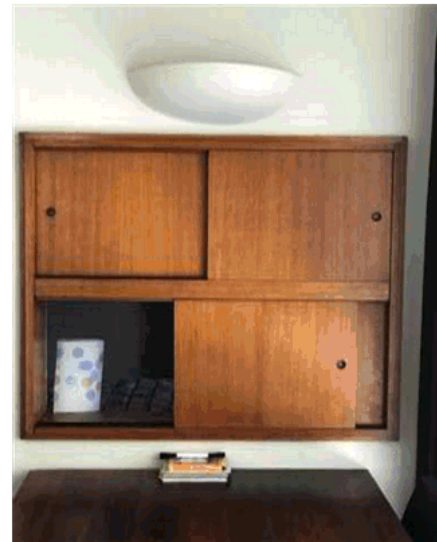
Figure 35. The maisonette (apartment 5) has a light coloured timber veneer sliding door servery unit between the kitchen and the dining nook. (Author photo)
