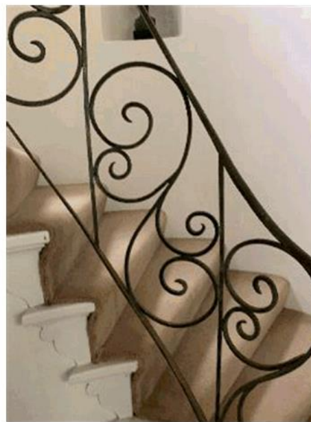
Figure 40: Main stair decorative wrought-iron balustrade.
