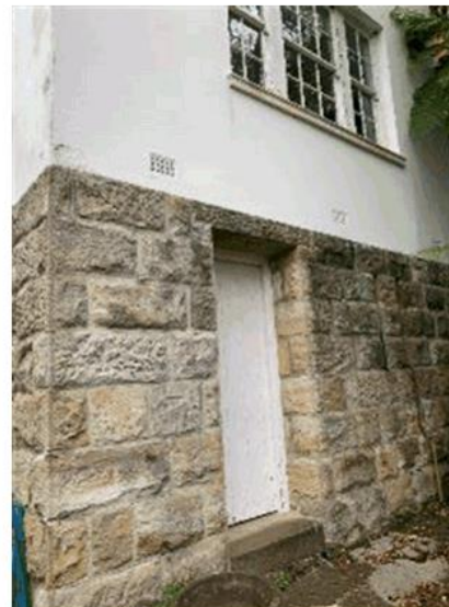
Figure 78: Sandstone base is generally in good condition.
