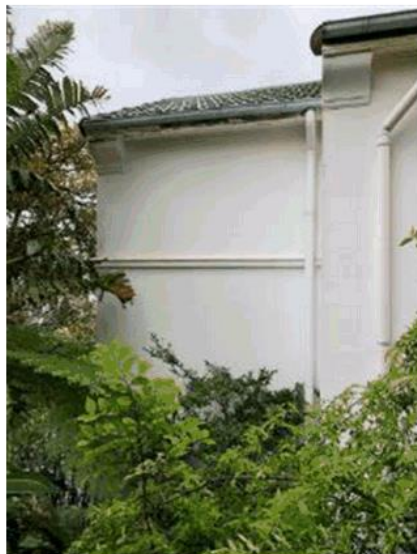
Figure 77: View of damage to eaves likely from gutter failure/overflow.
