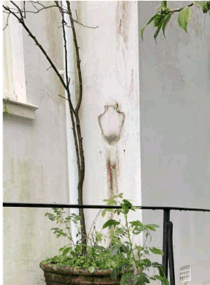
Figure 33: Rust staining and biological growth on the external wall
