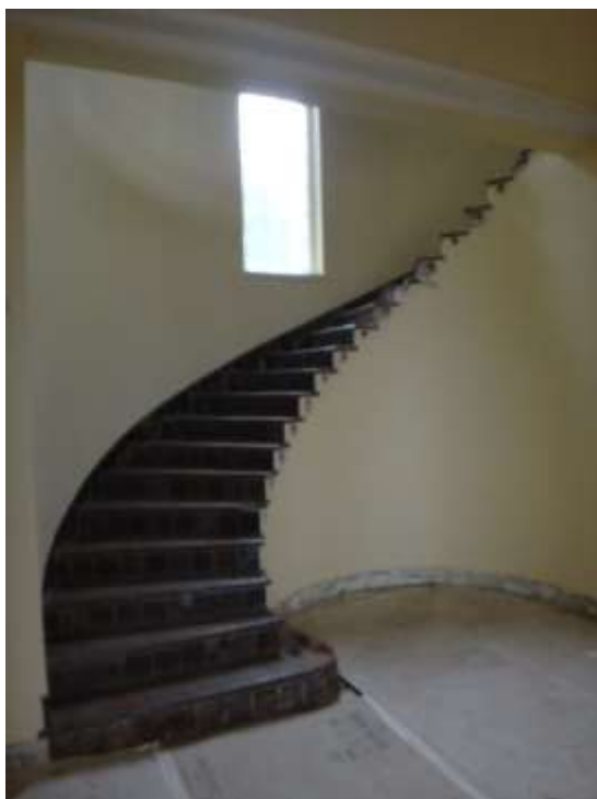
Figure 85: Main curved stair, with wrought-iron balustrade removed. The stair treads and risers are clad in stoneware tiles.
