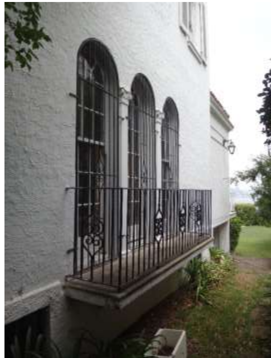
Figure 63: Northern elevation ground floor level arched openings to formal dining room, balconette and wrought iron balustrade.
