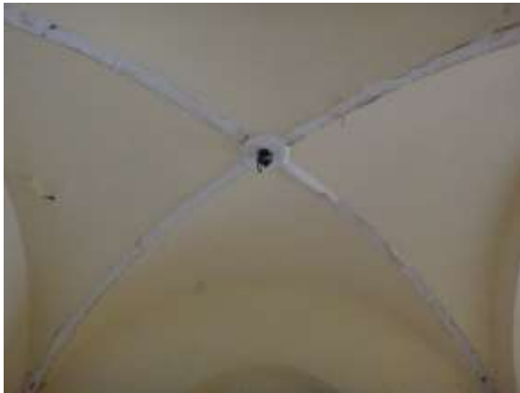
Figure 73: Vaulted ceiling to entryway. Evidence of decoration to ribs of the vaulted ceiling having been removed.
