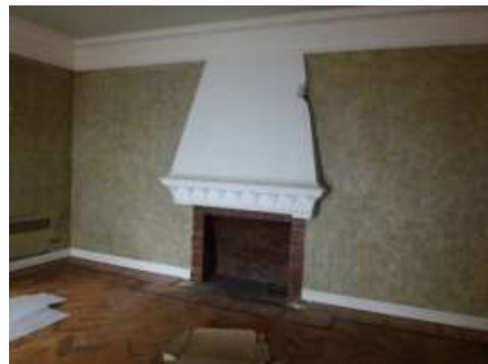
Figure 70: Fireplace as at 24 January 2020, with columns removed and minor damage to the hood.
