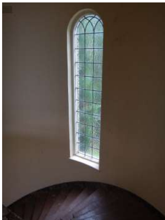
Figure 88: Arched window to the main stairs, with pointed glazing bars.
