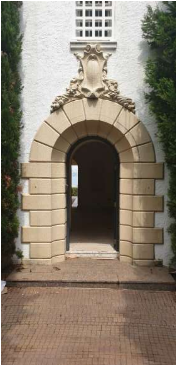
Figure 49: Decorative main entry on the front elevation with synthetic stone detailing, and window opening with grille above.
