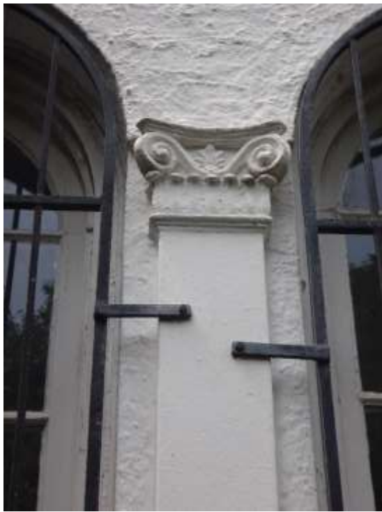
Figure 65: Detail view of pilaster to arched window openings
