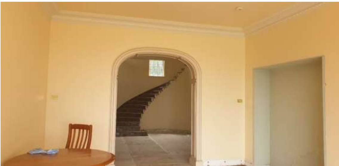
Figure 81: Looking back through the decorative archway to the main stair, which has had its balustrade removed. Some skirting has also been removed in this space.
