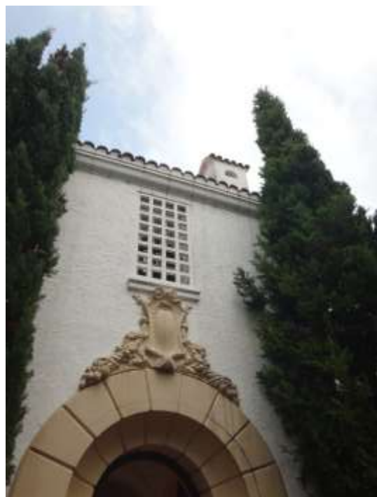
Figure 54: Decorative detail to arched entry, grille to bathroom window and tiled chimney crown visible above.
