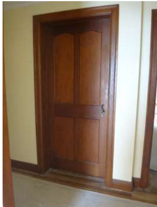
Figure 90: Detail view of timber door, skirting and architraves.
