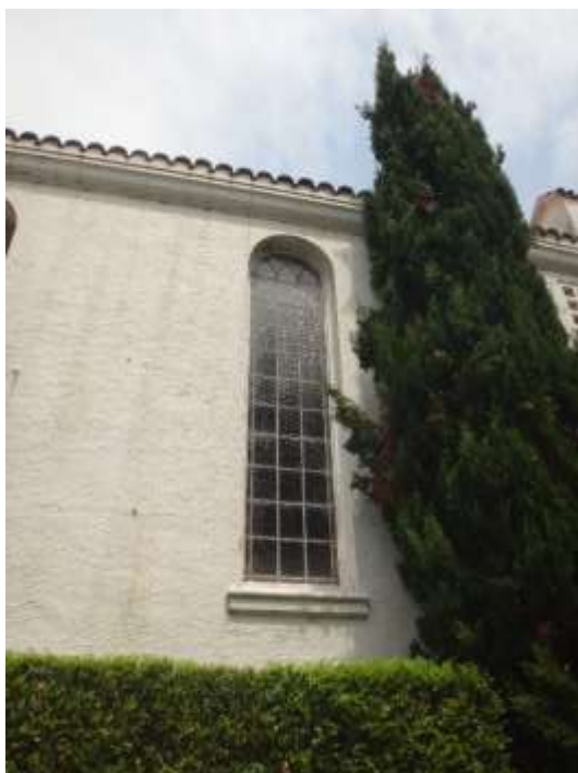
Figure 53: Arched window with pointed glazing bars to main stairwell.
