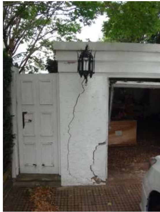
Figure 66: 1960s garage to the northern side setback showing substantial cracking.
