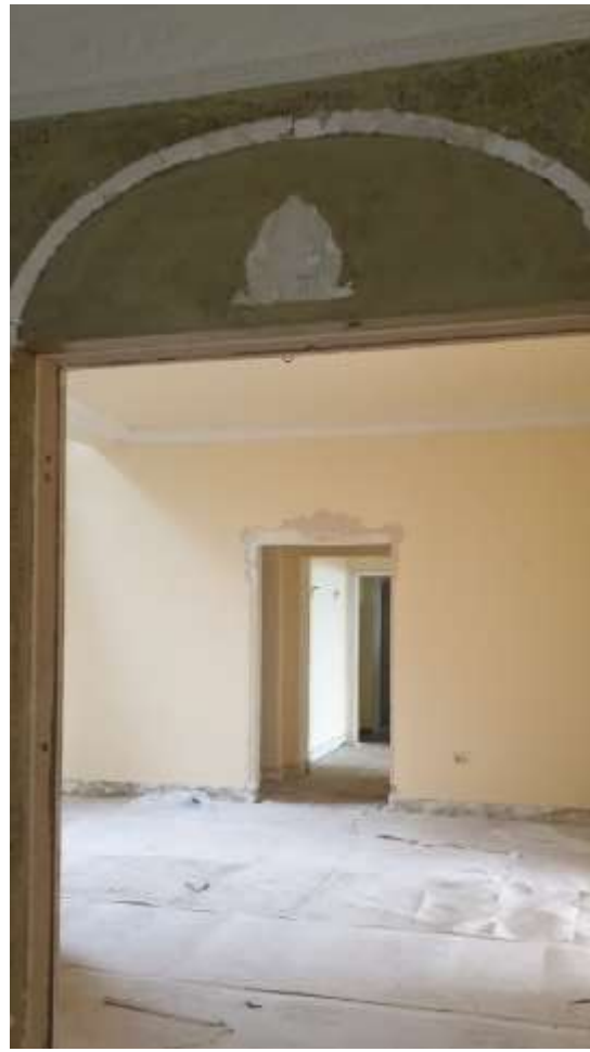
Figure 80: Opening from the former ballroom to entry hall showing decorative elements removed.
