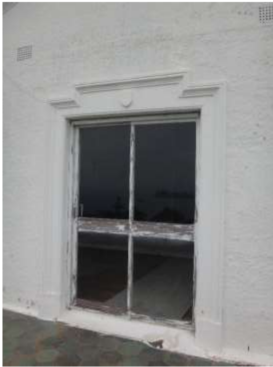
Figure 58: First floor rear elevation opening with wooden sliding door. This element originally featured a balconette.
