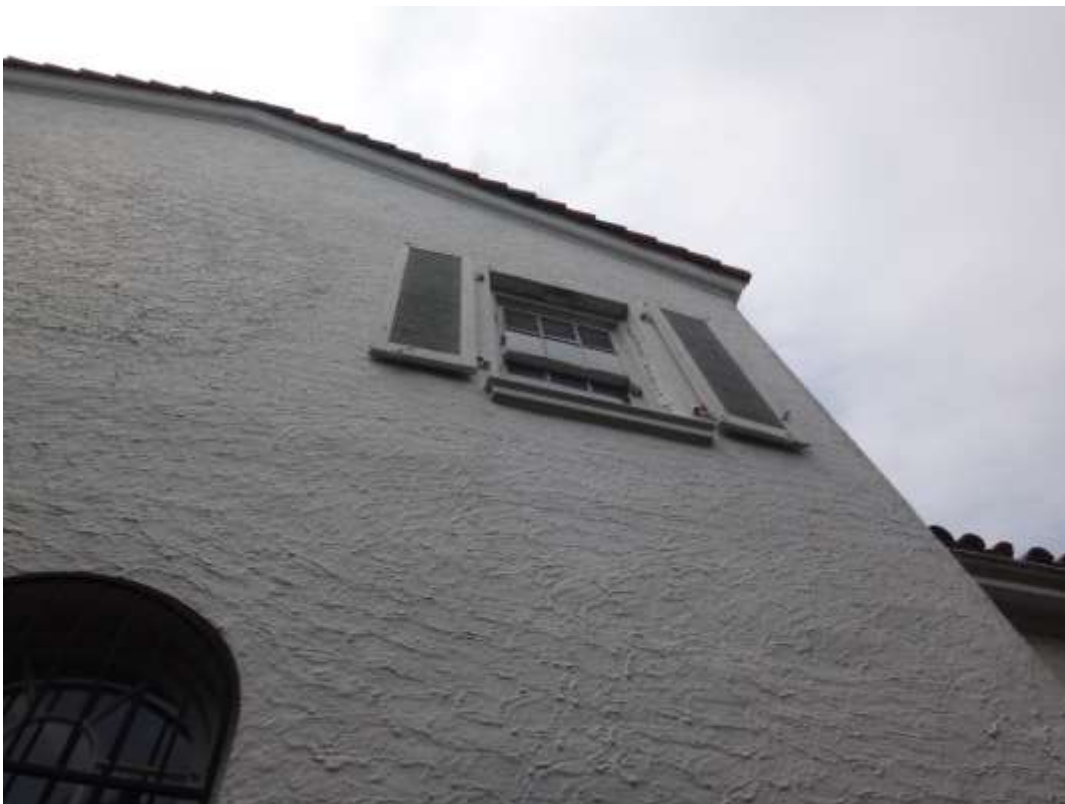
Figure 64: Northern elevation showing lightly textured rendering and first floor level 6 + 6 window opening with shutters.
