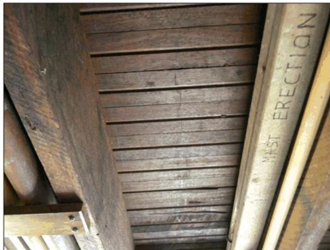
Figure 24: Floor joists and flooring (looking up to the first floor).
