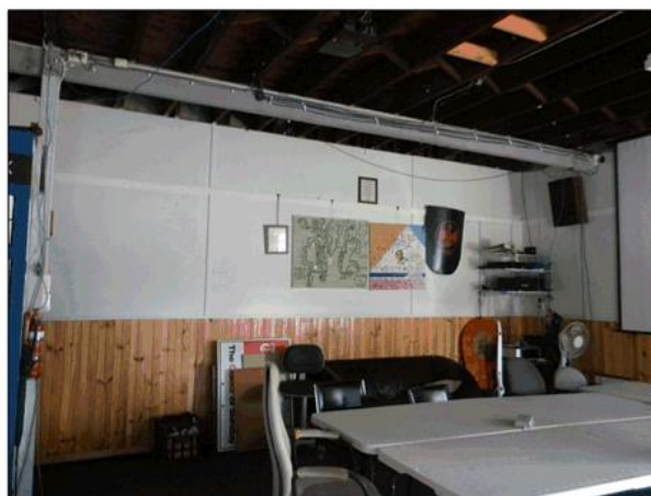
Figure 32: Partition wall, which does not reach to the ceiling.
