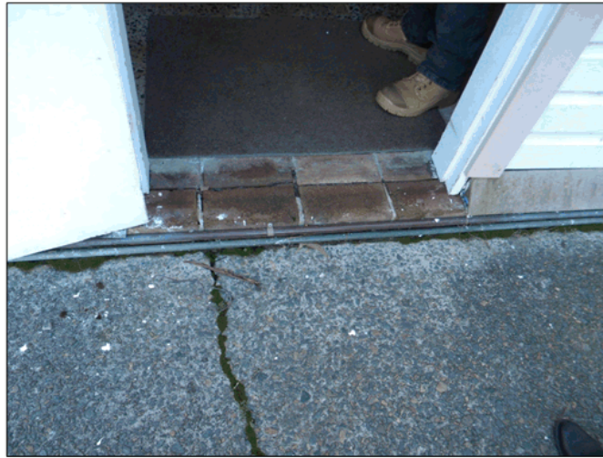
Figure 17: Brick threshold ground floor door.
