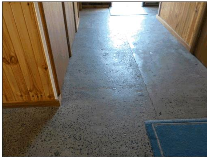
Figure 23: Concrete floor and vertical timber panelling.
