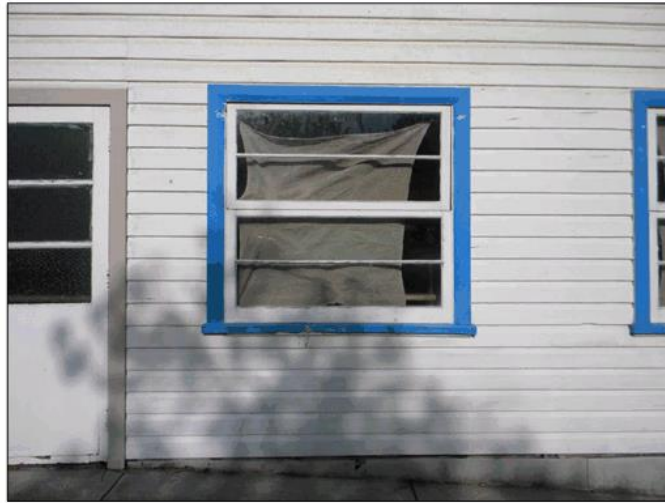
Figure 19: Detail of the awning sash windows.
