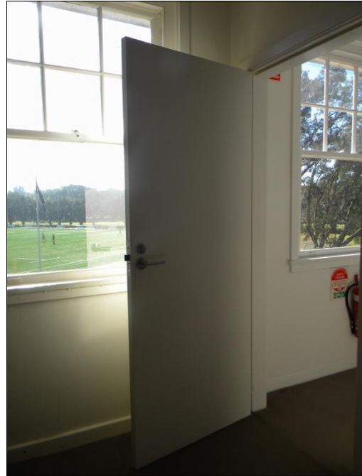
Figure 77: Showing simple finishes, typical at this level. Unprofiled skirting boards, simply detailed door and window architraves and single panel doors.
