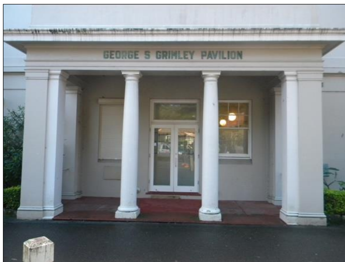
Figure 31: Entrance porch with red concrete floor.
