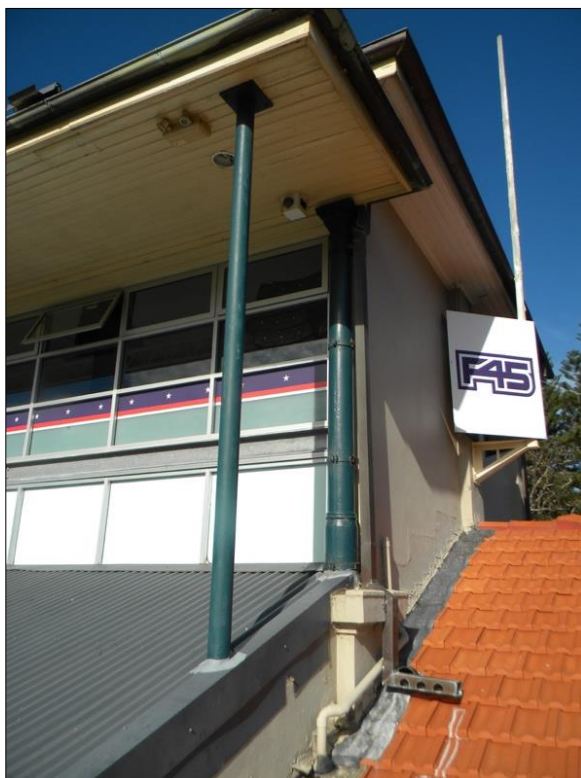
Figure 38: Posts supporting the roof.
