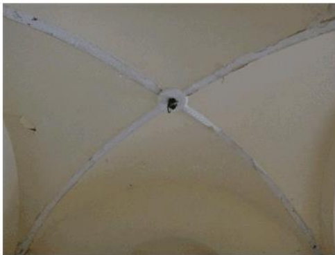
Figure 71: Vaulted ceiling to entryway. Evidence of decoration to ribs of the vaulted ceiling having been removed.
