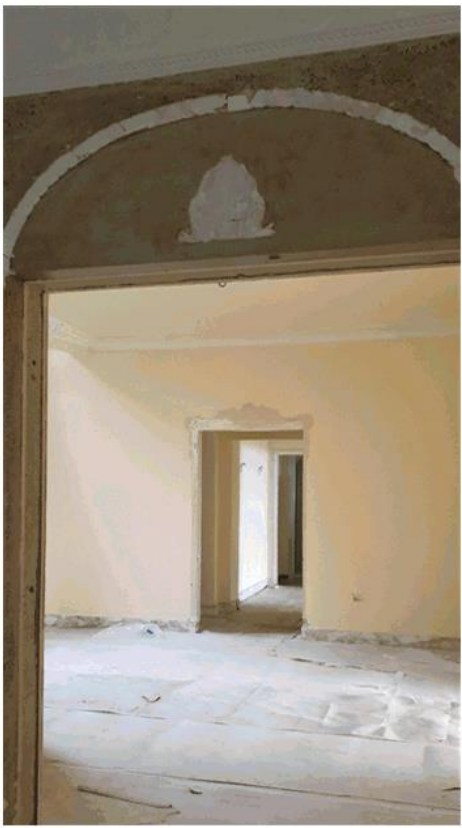
Figure 78: Opening from the former ballroom to entry hall showing decorative elements removed.
