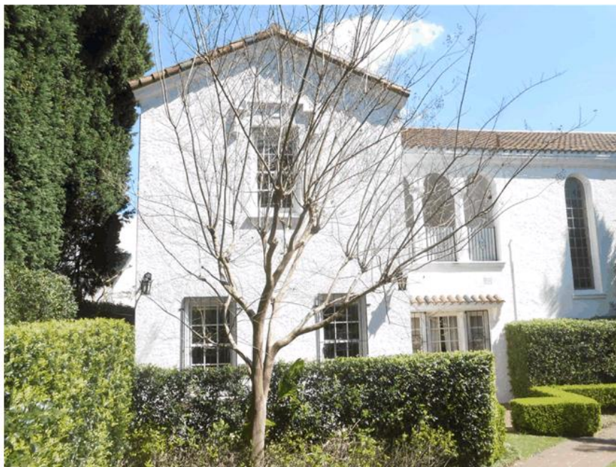
Figure 44: Gable end element on the front (Vaucluse Road) elevation with original pantiles and 6+6 timber windows. The first floor level opening has moulded decoration above. The first floor level sleepout with decorative columns and the arched leadlight opening to the main stair are also visible. (Source: WMC Officer, 2015)
