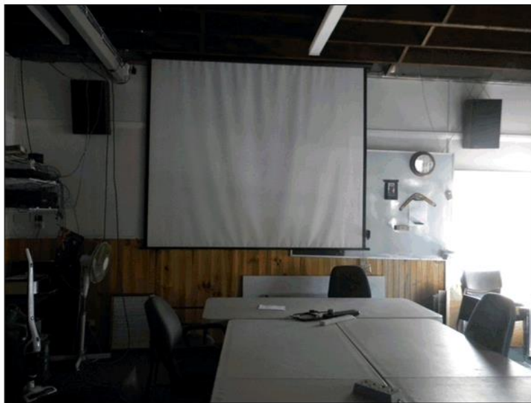
Figure 31: First floor, with vertical timber panelling and plasterboard/fibro-lined walls with cover strips. There is no ceiling, exposing the roof above.
