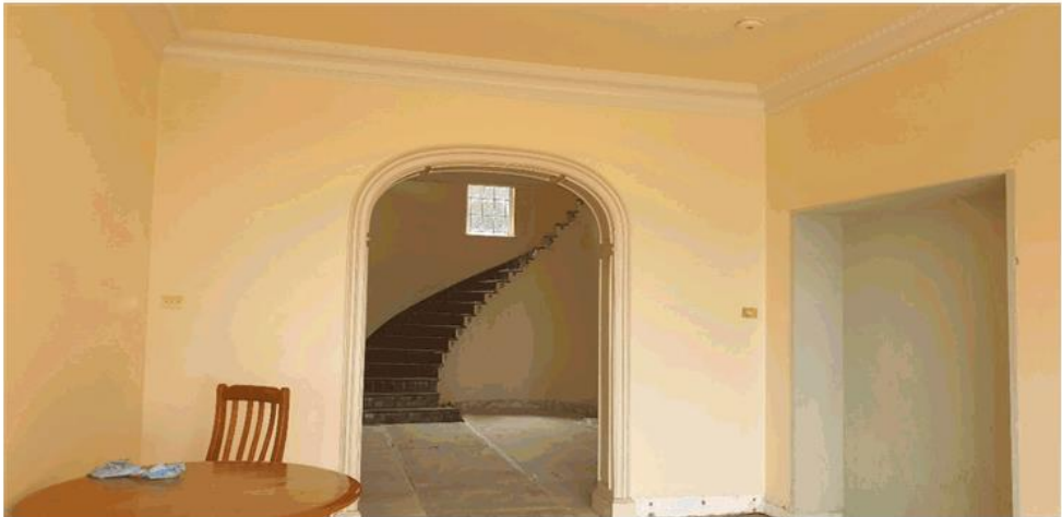
Figure 79: Looking back through the decorative archway to the main stair, which has had its balustrade removed. Some skirting has also been removed in this space.
