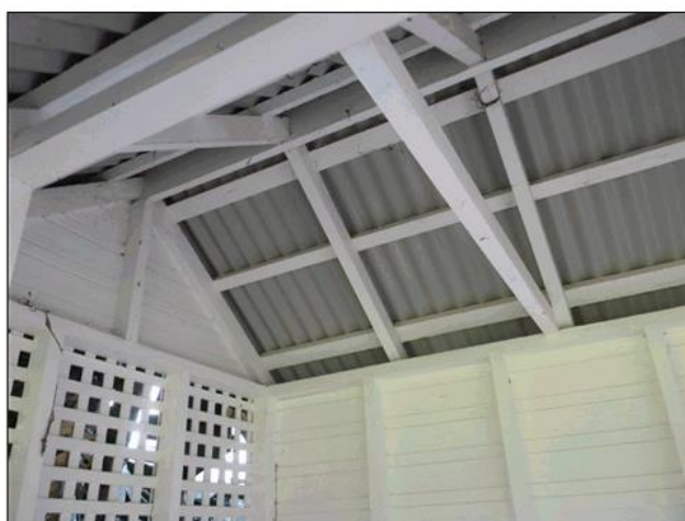
Figure 56: Timber roof framing.
