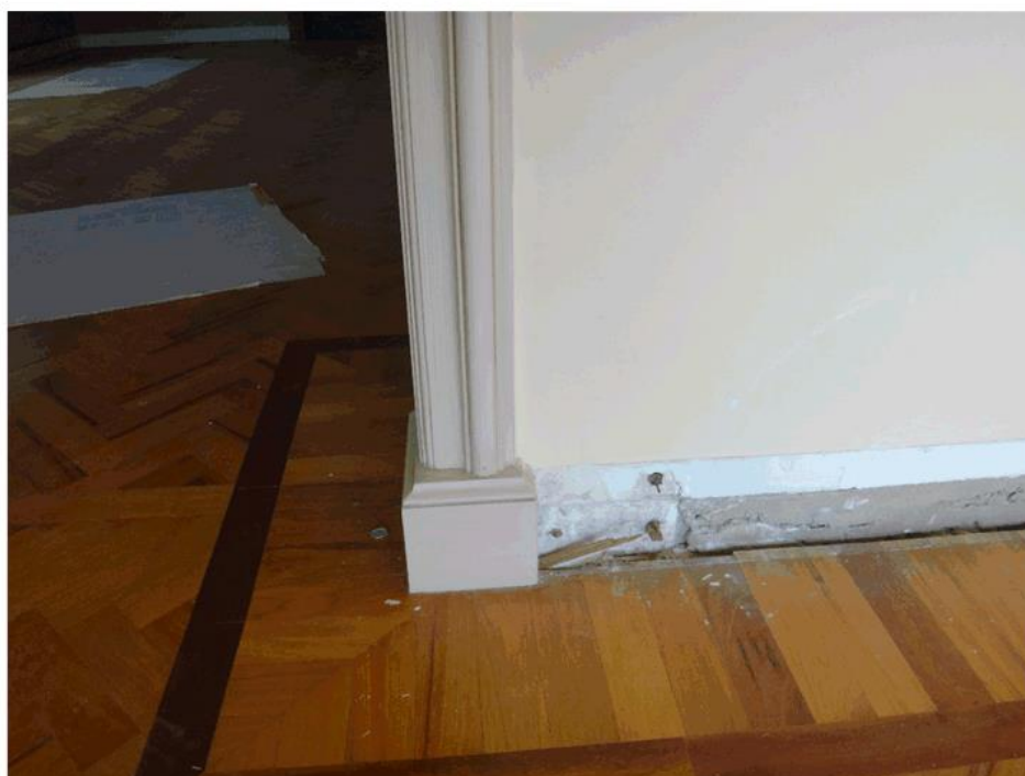
Figure 74: Decorative skirting and architraves have been partially removed. Herringbone parquet flooring remains to the formal dining and former ballroom.
