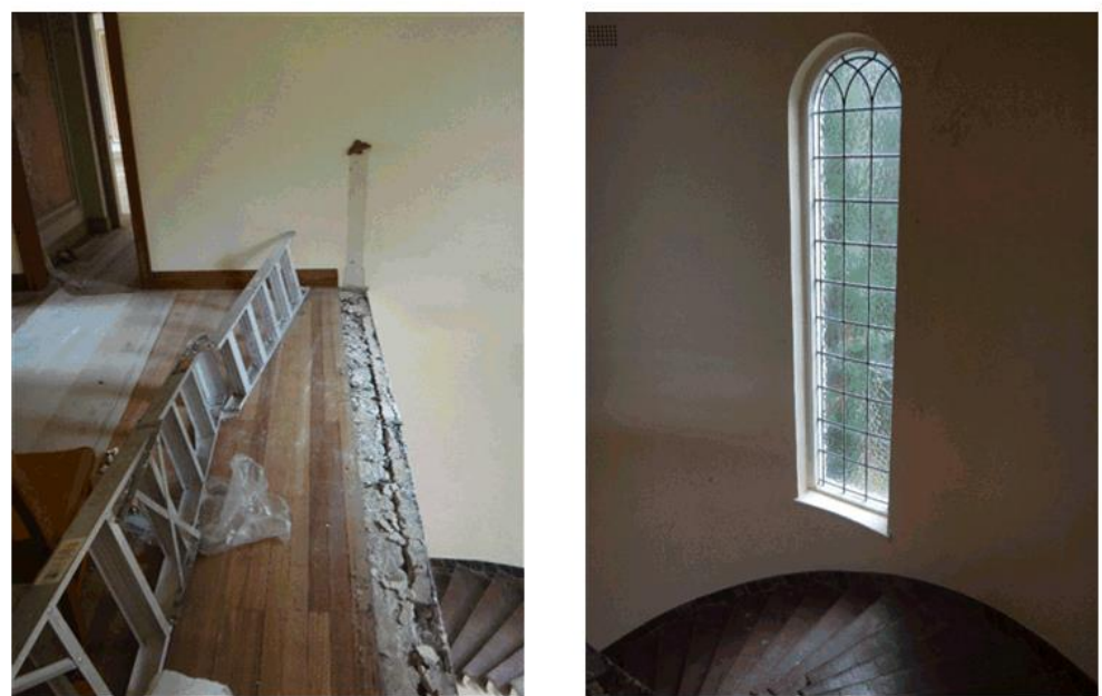
Figure 85: Balustrade to the first floor level landing has been removed
