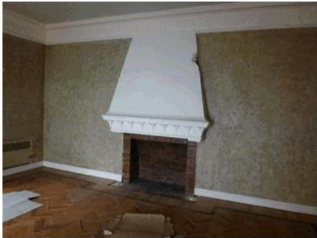
Figure 68: Fireplace as at 24 January 2020, with columns removed and minor damage to the hood.
