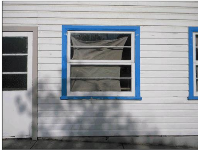
Figure 19: Detail of the awning sash windows.
