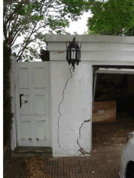
Figure 64: 1960s garage to the northern side setback showing substantial cracking.
