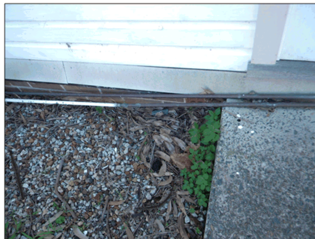
Figure 57: Repair where a lower weatherboard has rotted out.
