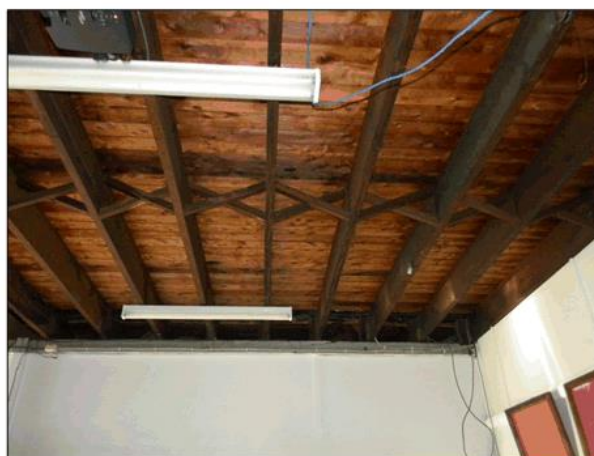
Figure 34: Exposed rafters.
