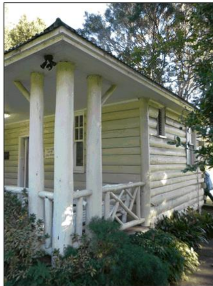
Figure 33: Detail of the rough timber posts supporting the roof.
