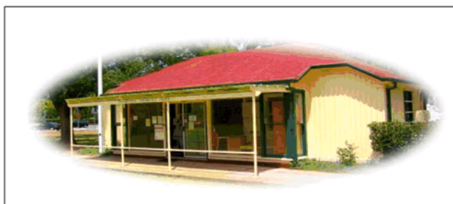
Figure 66: Williamstown Croquet Club. Google Images Fibre-cement sheet and battening.
