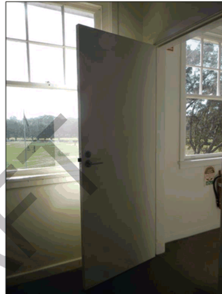
Figure 72: Showing simple finishes, typical at this level. Unprofiled skirting boards, simply detailed door and window architraves and single panel doors.
