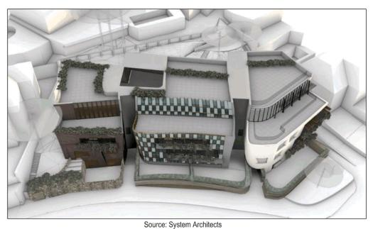
Figure 4: Bird's eye view of the building showing Level 3 setback behind the front facade
