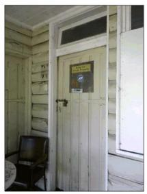
Figure 41: Single door with top light into the main part of the building.
