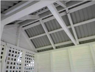
Figure 56: Timber roof framing.
