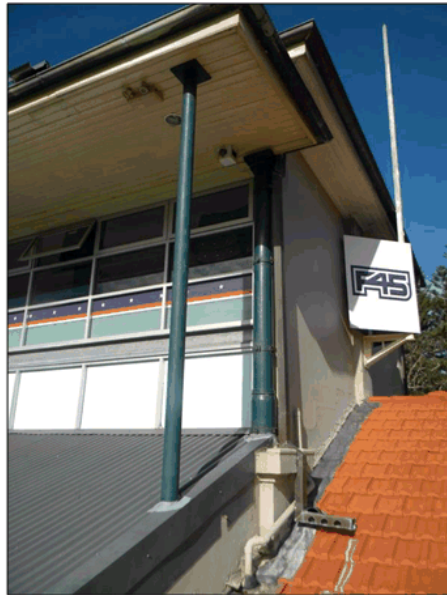
Figure 38: Posts supporting the roof.
