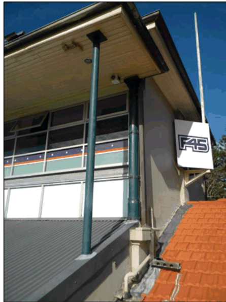
Figure 38: Posts supporting the roof.
