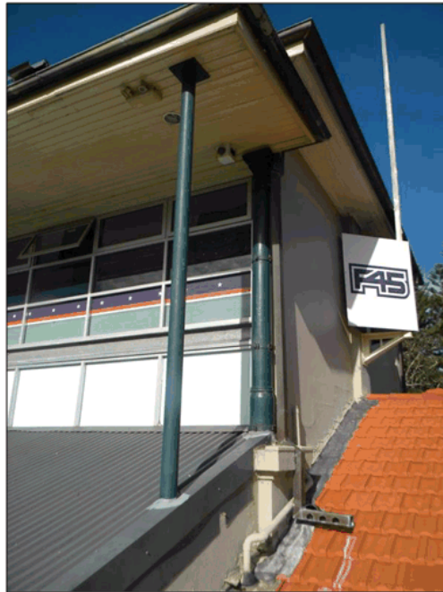
Figure 38: Posts supporting the roof.
