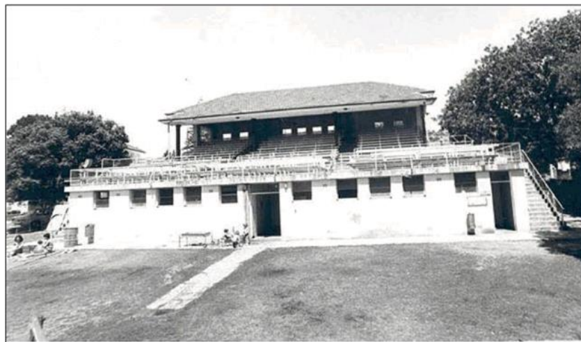
Figure 15: The north-eastern elevation of the George S. Grimley Pavilion in 1978. Note seating, since replaced with a flat deck and, at the top of the grandstand, beneath the tiled roof, an enclosed gymnasium.
