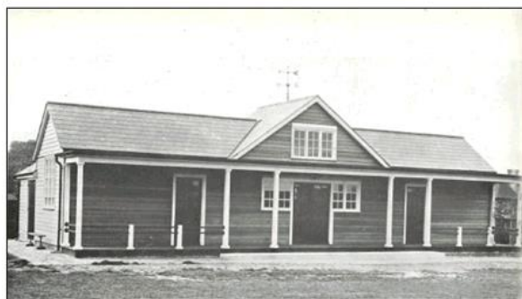
Figure 17: Pavilion at the Canterbury Simon Langton School for Girls (England). This building is of timber construction, the walls being covered with cedar weatherboarding. Accommodation; two changing rooms, a large tea-room, kitchen and stores. Timber Buildings for the Country, 1938.
