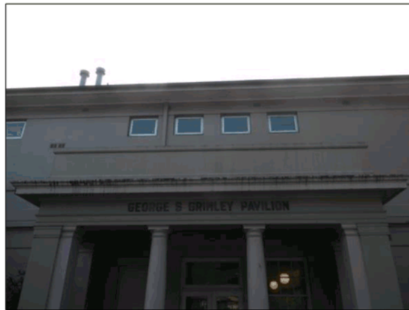
Figure 30: Detail of the metal framed highlight windows at first floor level.
