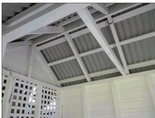
Figure 56: Timber roof framing.
