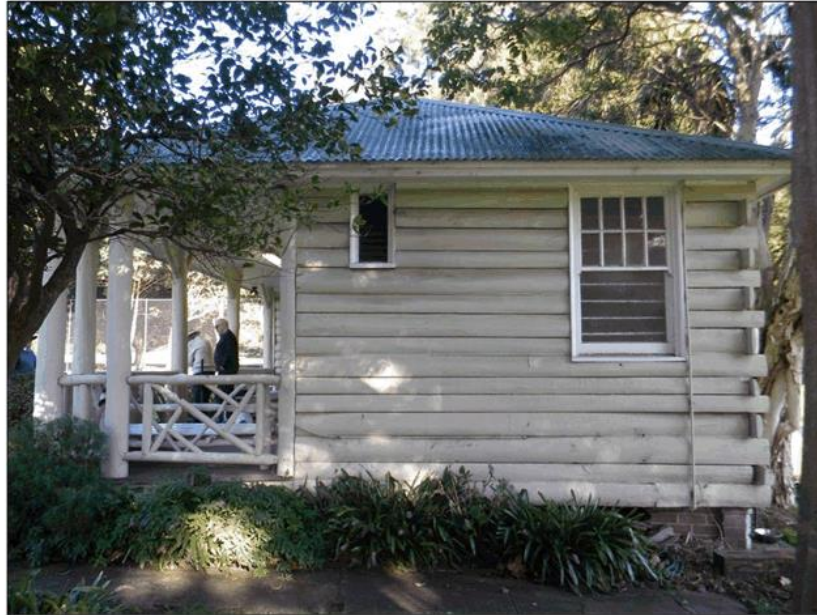
Figure 34: Detail of the rough timber posts supporting the roof.
