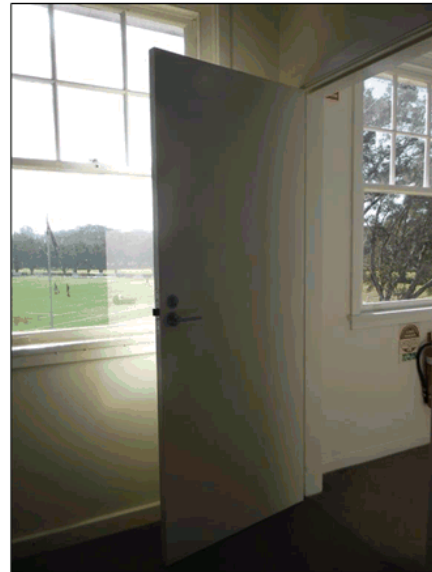
Figure 77: Showing simple finishes, typical at this level. Unprofiled skirting boards, simply detailed door and window architraves and single panel doors.
