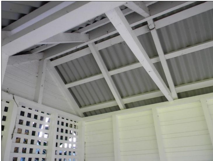
Figure 56: Timber roof framing.
