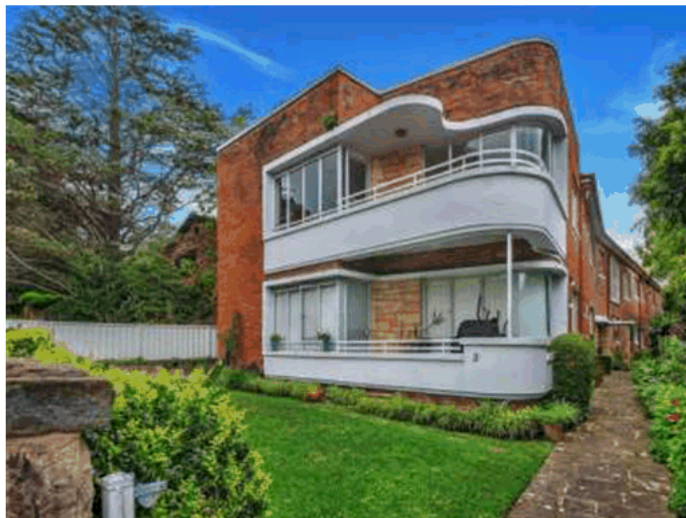
Figure 15. Trelawney Court viewed from Trelawney Street east; note distinctive “S” shaped first floor concrete awning slab edge- and curved sandstone feature panels. Sandstone flagged path leads to lobby entry. (Source: Bradfield Cleary 2019)
