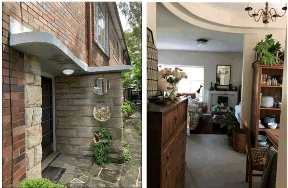
Figure 5 and 6: Main entry door with a curve concrete slab awning over an ashlar sandstone blade wall and curved 'streamlined' plasterwork.
