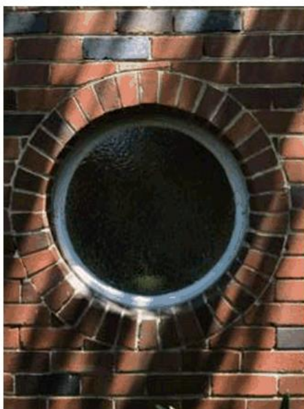
Figure 26. The building has many types of steel windows e.g. this pivoted porthole window to a WC. (Author photo)
