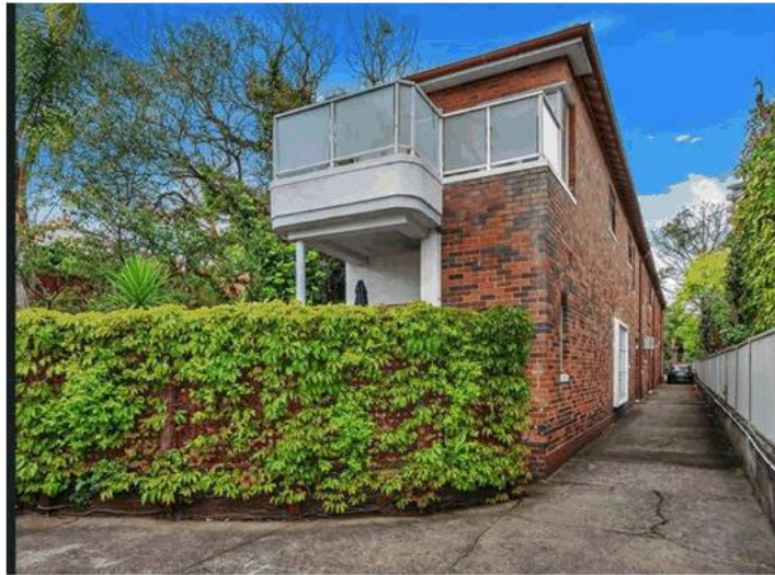
Figure 18. Trelawney Court viewed from north, rear (garage); detailing of curved rendered balustrade panels has been repeated to compose a formal garden facade. Intrusive pool fence type balustrade has been added recently. (Source: Bradfield Cleary 2019)
