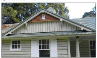
Figure 27: Detail of the southfacing gable, showing terracotta shingles, vent and split log.
