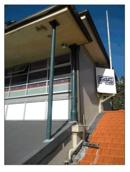
Figure 38: Posts supporting the roof.
