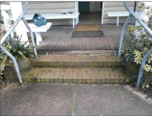
Figure 29: Brick stairs with pipe rail balustrade leading up to the entrance at the eastern end.
