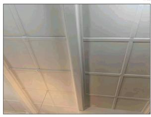
Figure 45: Detail of the ceiling with bearers and battening. One section has a small plaster detail at the point where the battens cross (LHS). This detail is absent on the other section (RHS).
