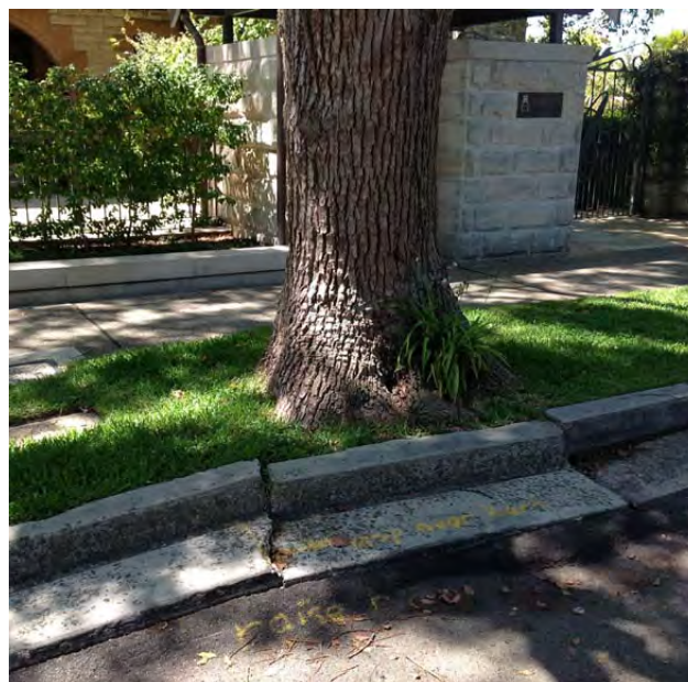
Figure 1.10 -Infrastructure damage is one of the most common impacts of street tree planting (Photo Arterra)
