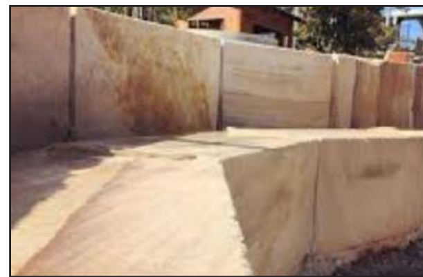
SANDSTONE RETAINING WALL
