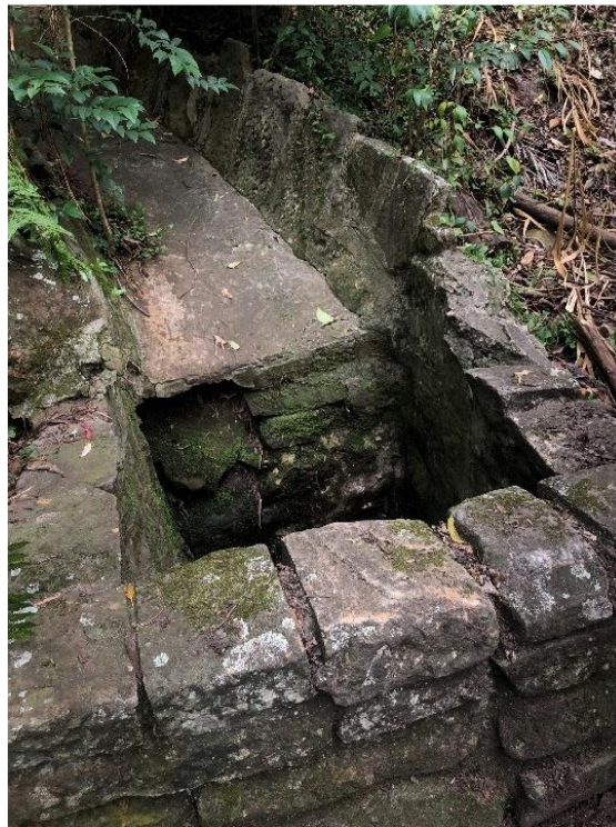
Figure 21 Original or early sandstone drainage channel and pit, Cooper Park. (Photo: Chris Betteridge, 29 March 2019)
